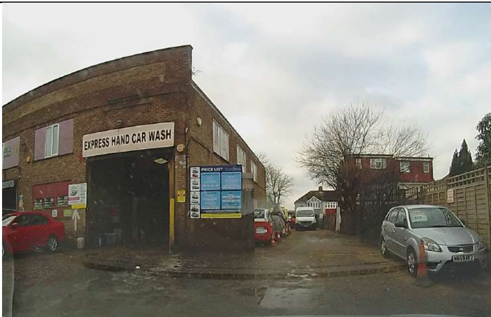
Photo 2: Image looking west along northern boundary.
