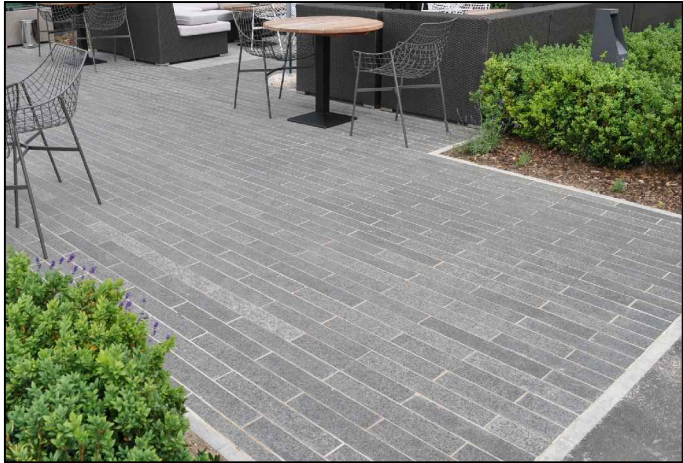
Plank type granite paving
