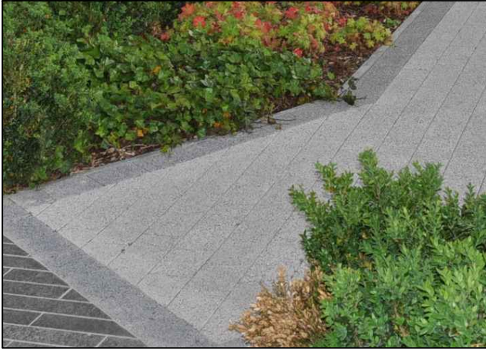
Plank type granite paving
