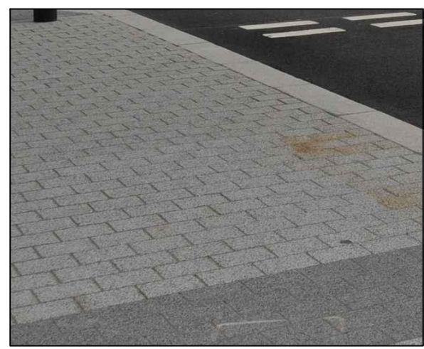
Granite paving in contrasting colours
