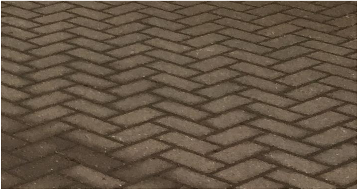
Existing garage courtyard block paving (relatively new)
