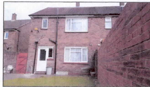
VIEW OF REAR ELEVATION FROM BACK GARDEN
