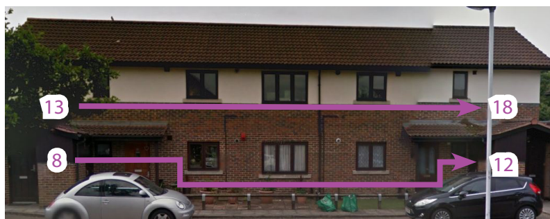
Assessed windows on the north facade of 20-21 Farrier Close
