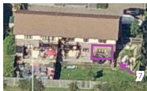
Assessed windows on the south facade of 20-21 Farrier Close
