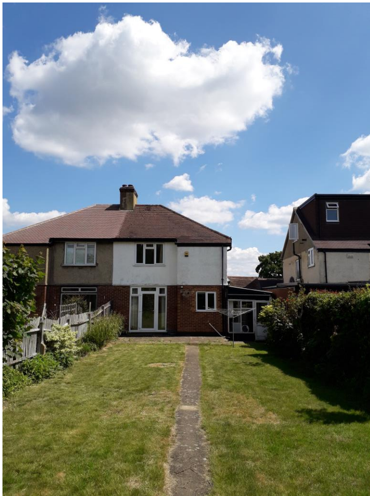
Fig.1 Photo showing of existing property to rear
