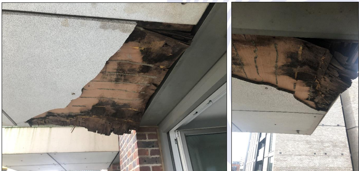
Figure 1.1: Image showing the degraded balcony soffits.
