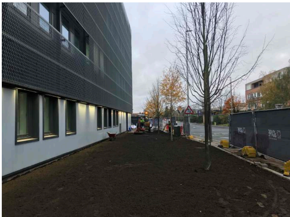
Photo 2 Top soil complete to Blyth Road planting area
