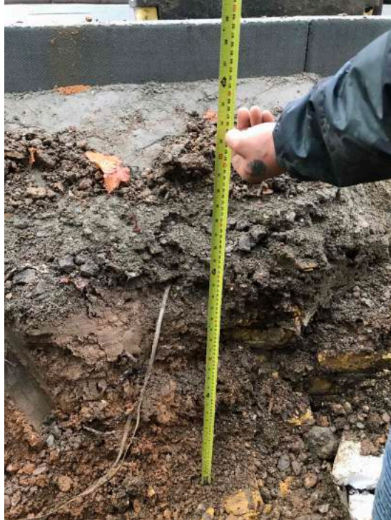
Photo 7 Tree pit section along blyth road, dug out ahead of sub soil
