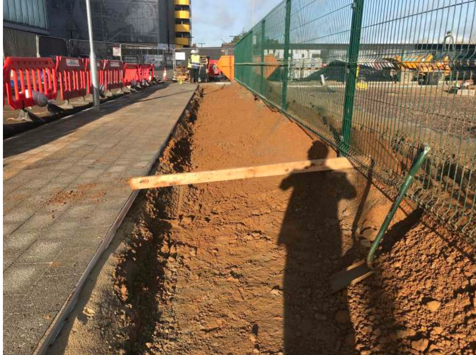
Photo 21 Sub soil installed to south elevation planting section leaving 350mm for top soil and bark mulch
