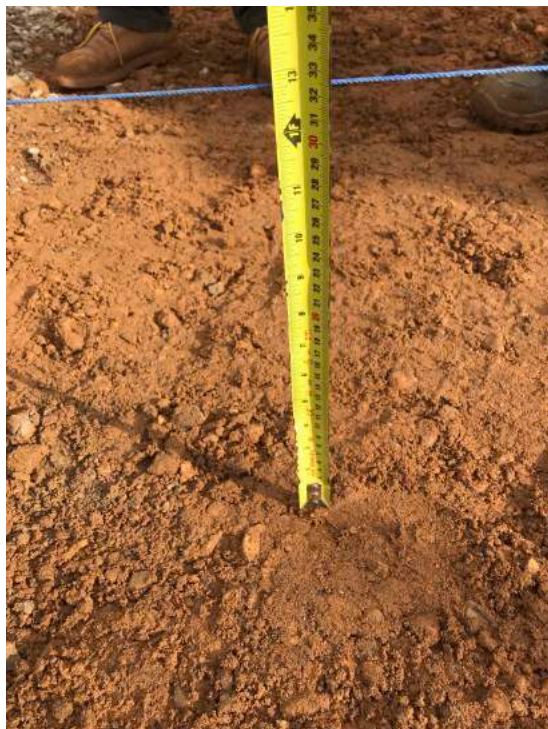
Photo 12 Sub soil installed ahead of top soil to tree pit and planting section next to sib station - South elevation
