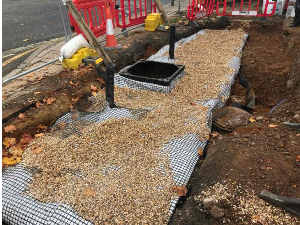
Photo 23 Mesh terram to top of tree crates in hard landscape ahead of back fill
