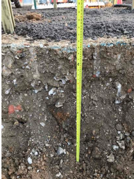
Photo 9 Tree pit next to bin store ahead of sub soil. 1m deep
