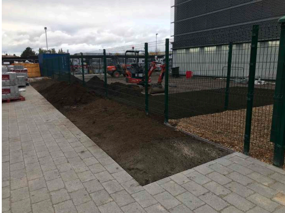
Photo 11 Top soil being installed to South elevation planting section either side of fence line
