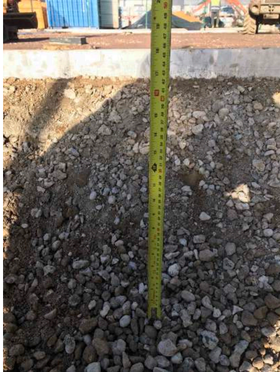
Photo 15 450mm depth for sub soil and top soil to planting section in courtyard next to sub station
