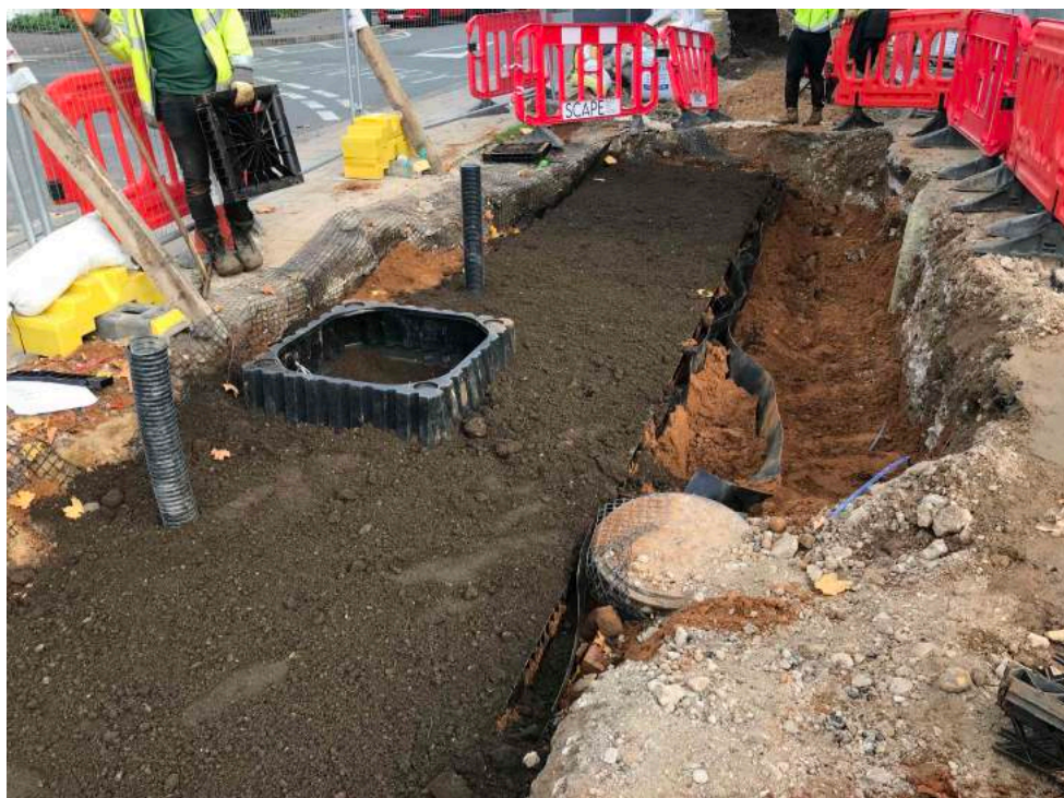
Photo 24 NW corner tree pit now top soiled
