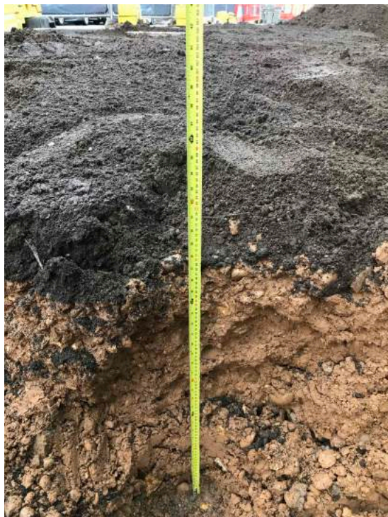
Photo 6 Sub soil and top soil being installed to the Blyth road tree section
