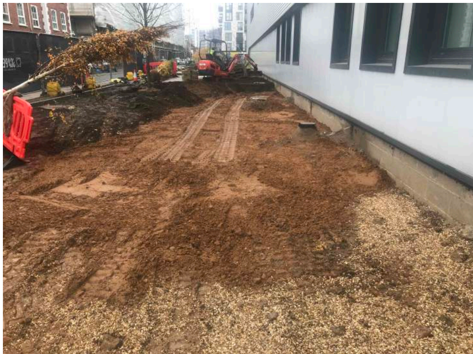
Photo 4 Sub soil being installed and initial top soil to blyth road large planting area
