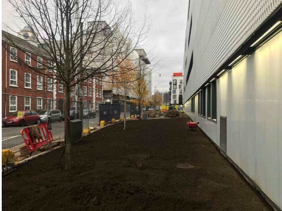
Photo 1 Top soil complete to blyth road planting section
