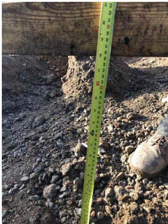
Photo 20 Planting section dug out either side of fence line along West elevation corner, nearer bin store end, ahead of sub soil
