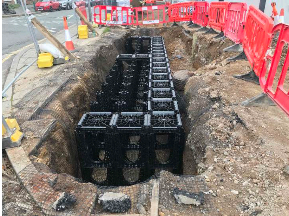
Photo 25 Tree pit crates being installed for hard landscaping tree pit NW corner
