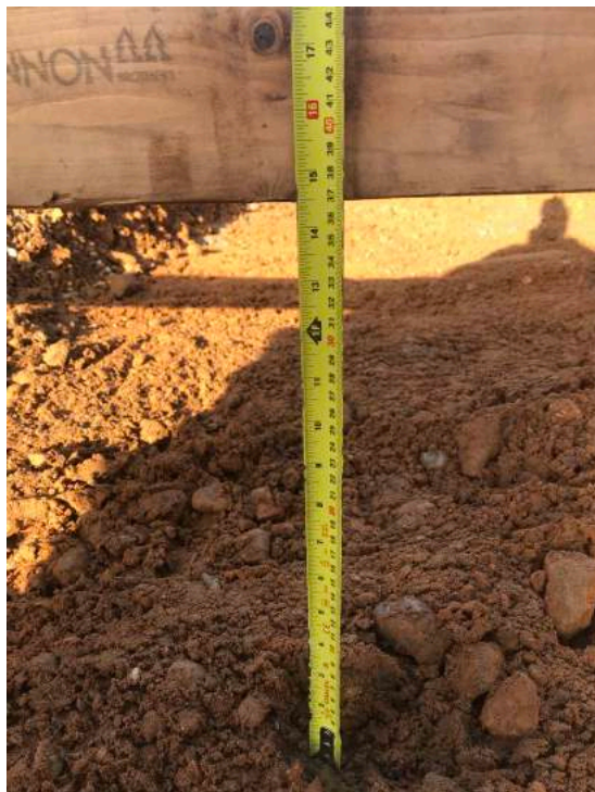
Photo 22 Sub soil installed to planting section next to fence line on West elevation allowing for 350mm topsoil and bark mulch
