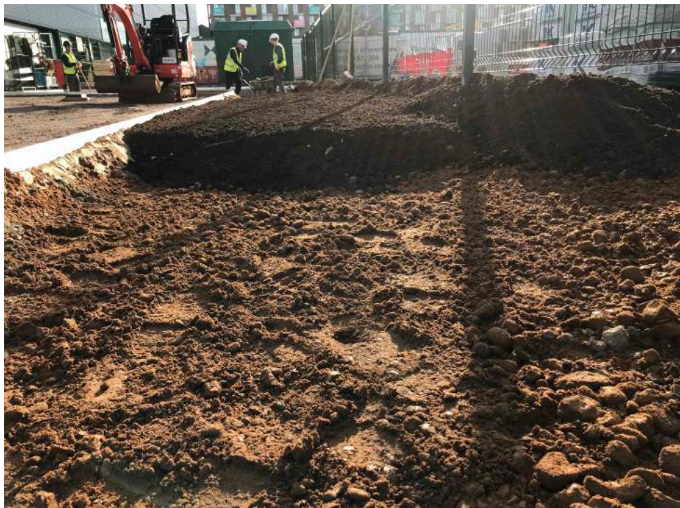
Photo 14 Top soil of minimum 300mm to planting and tree section in South courtyard
