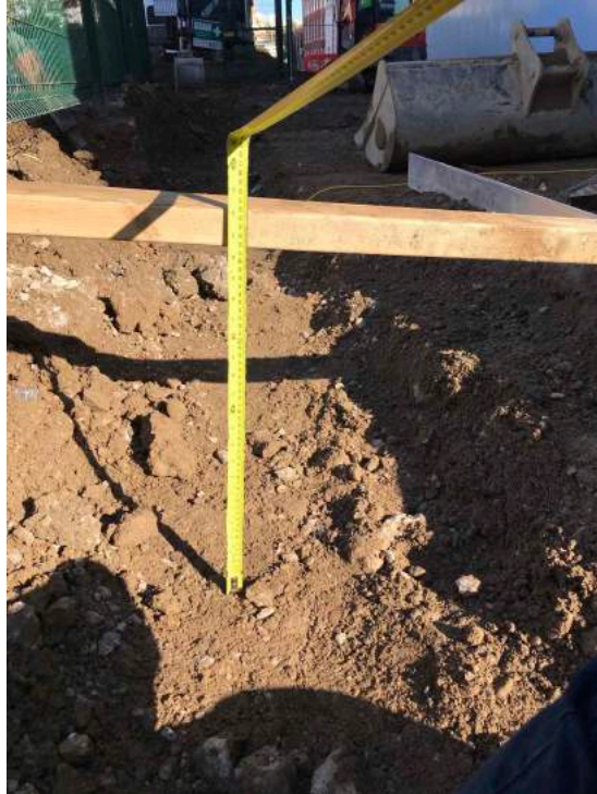
Photo 17 Trench dug to 500mm depth for planting section next to fence line on West elevation.
