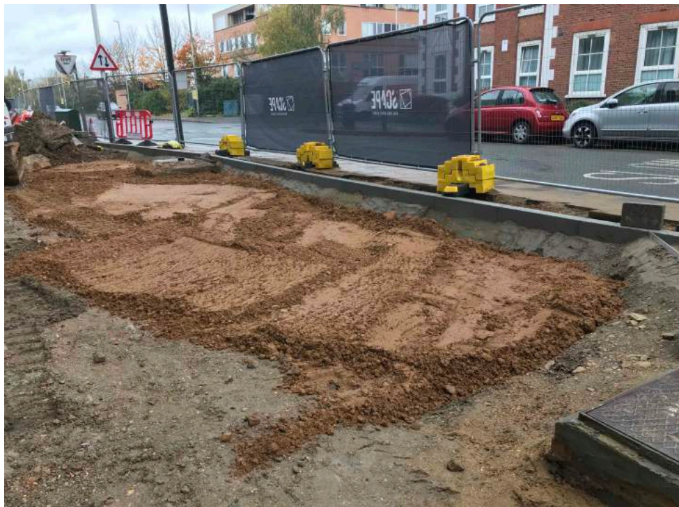
Photo 8 Sub soil complete to blyth road tree section ahead of top soil install
