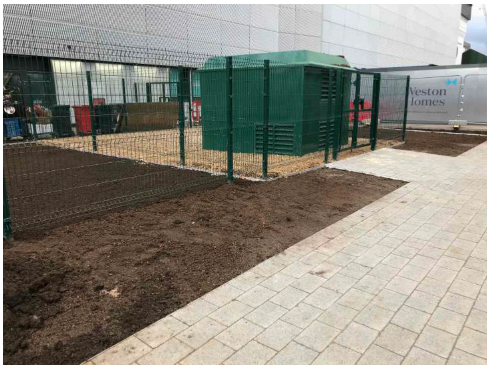
Photo 10 Top soil install to planting area next to fence line on south elevation
