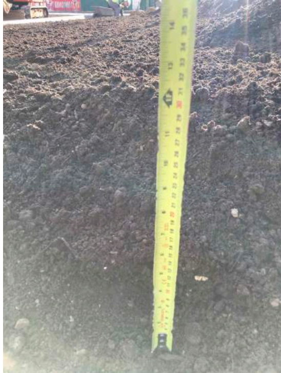
Photo 13 South elevation planting and tree section top soil depth
