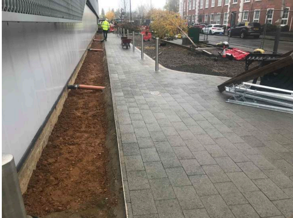
Photo 3 Sub soil to blyth road barrow planting section leaving 350mm for top soil and bark mulch
