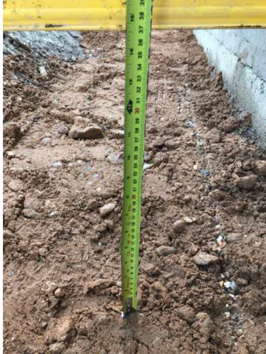
Photo 19 Sub soil laid - depth for top soil. Blyth road narrow section against building
