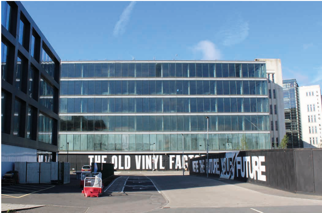
The Cabinet Building
