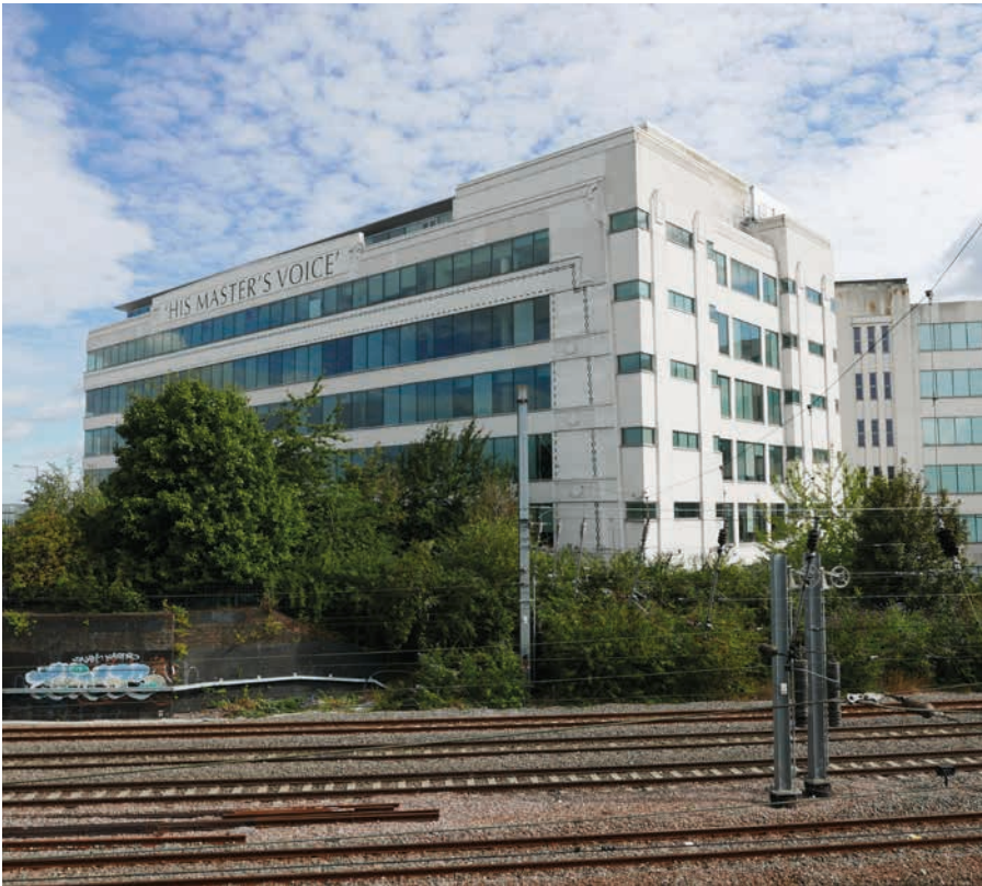
The Shipping Building
