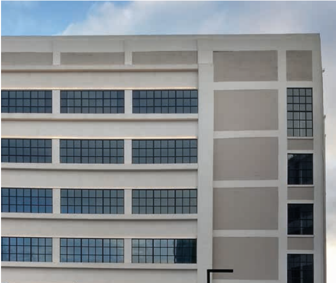
The Record Store presents a simple, repetitive facade
