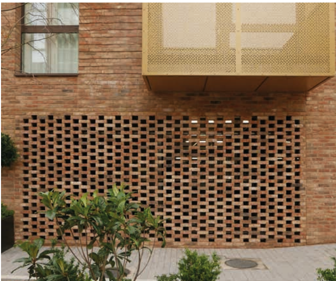
Hit and miss brickwork creates interest and ventilation to cycle stores
