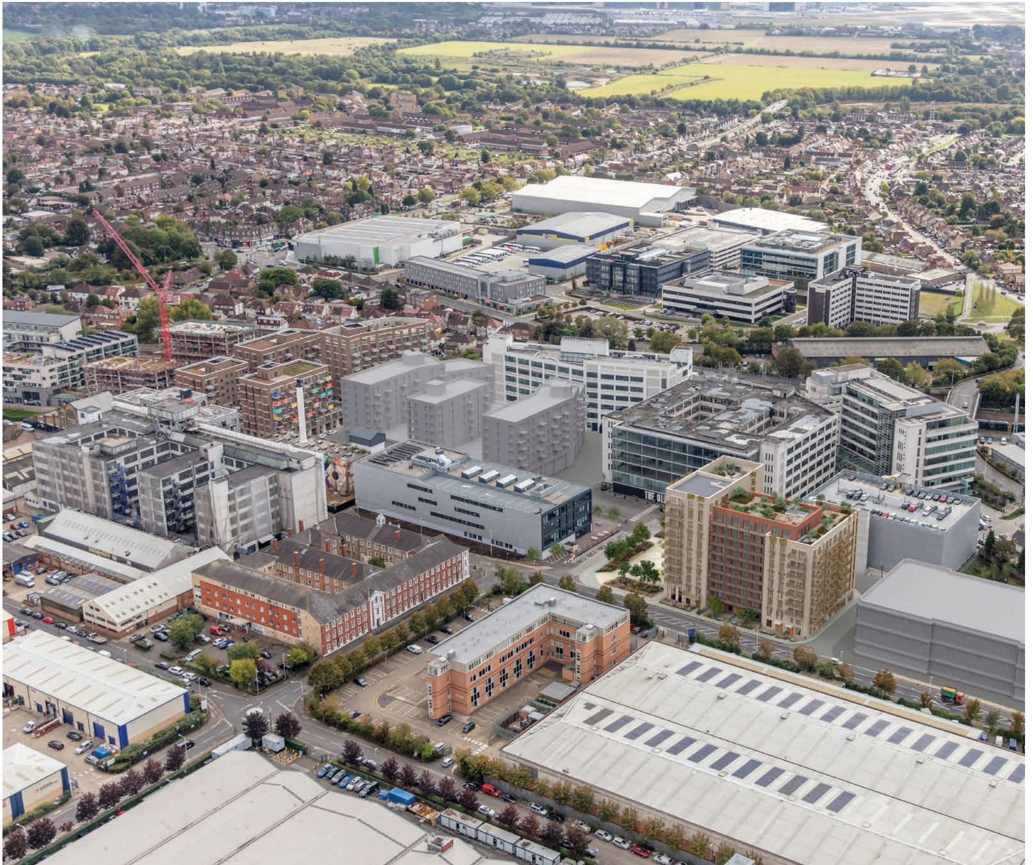
View looking south across The Old Vinyl Factory site
