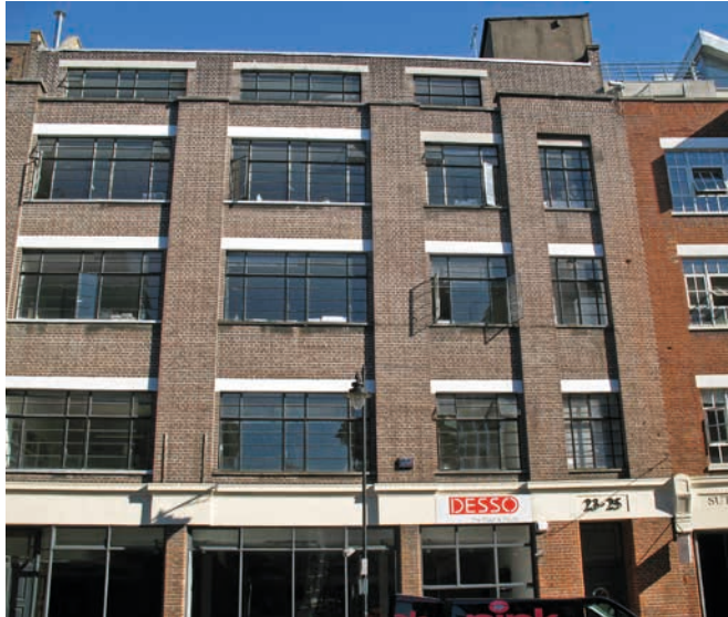
Traditional warehouse aesthetic with crittal windows in Clerkenwell, London
