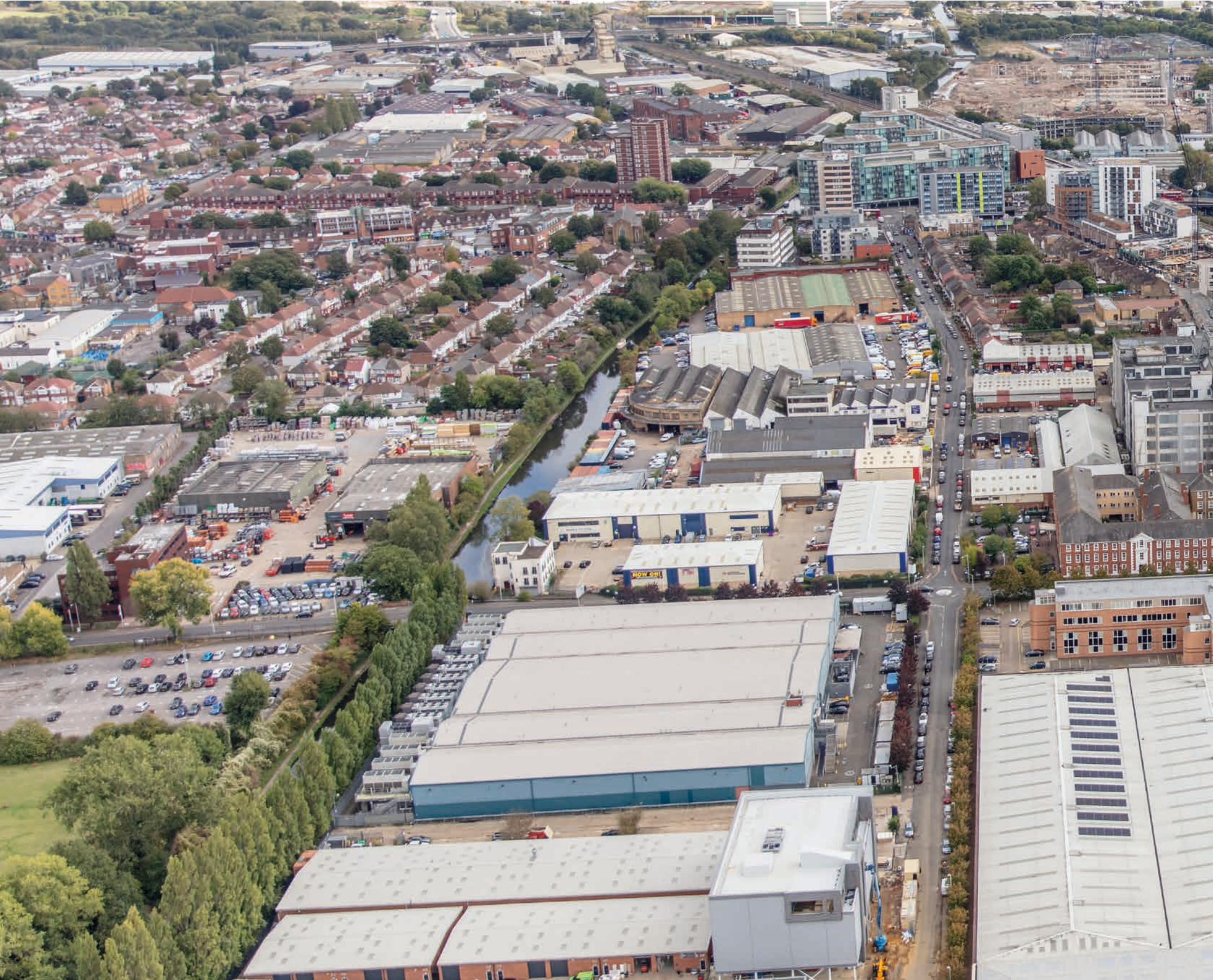
View looking east across The Old Vinyl Factory site towards Hayes Town Centre and station
