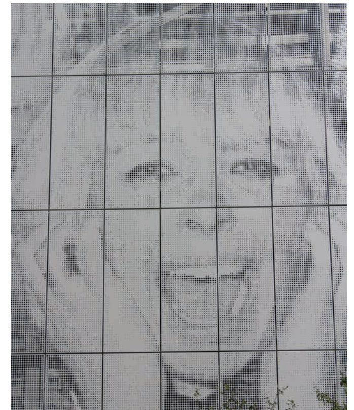
Metalwork detailing takes various forms at The Old Vinyl Factory
