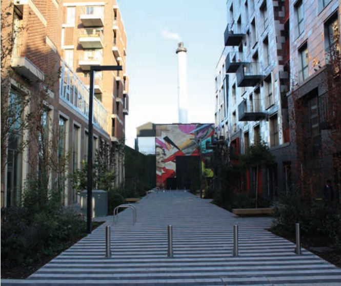
'The Groove' running between the Material Store and The Boiler House
