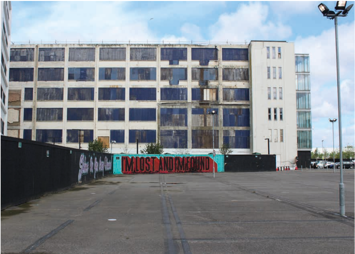
The Cabinet Building
