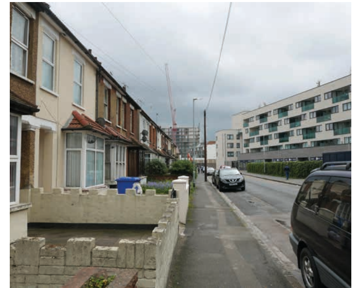
Blyth Road Victorian Housing with Gatefold Building beyond
