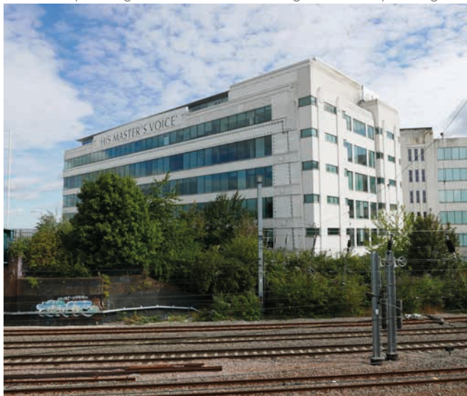
The Shipping Building
