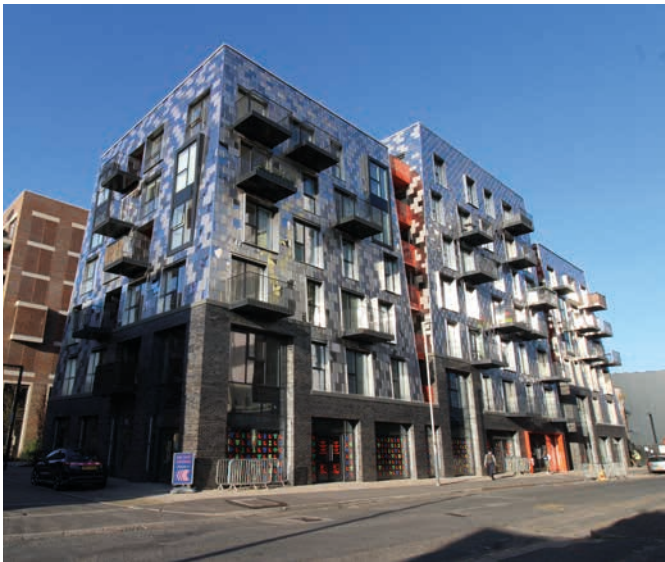
The Boiler House
