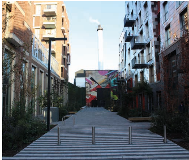
The Groove between the Material Store and The Boiler House
