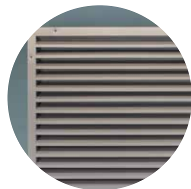
Concealed framed louvres used in new extension
