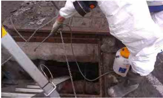
Spraying asbestos surfactant onto potential ACMs in duct prior to entry
