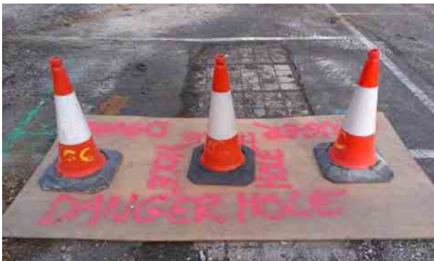
Warning and covers placed over access holes where original covers not be replaced
