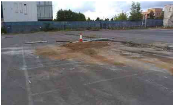
Typical trial pit reinstatement condition
