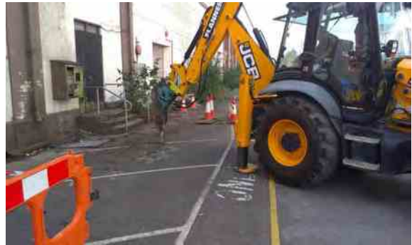
Removing access covers with aid of JCB
