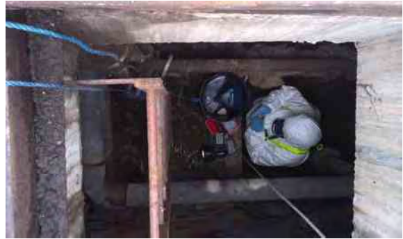
View into duct during surveying and sampling works
