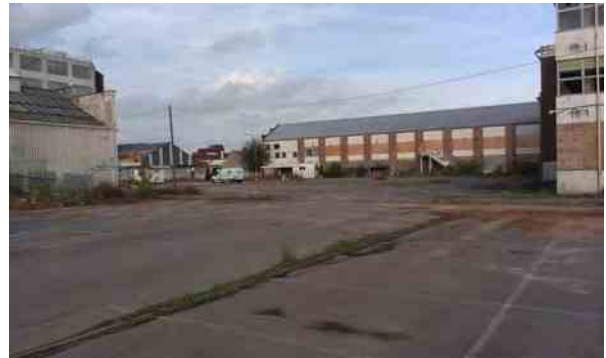
View towards Apollo House on completion Soilfix works
