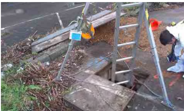
Lagged pipe housed in chicken wire in duct
