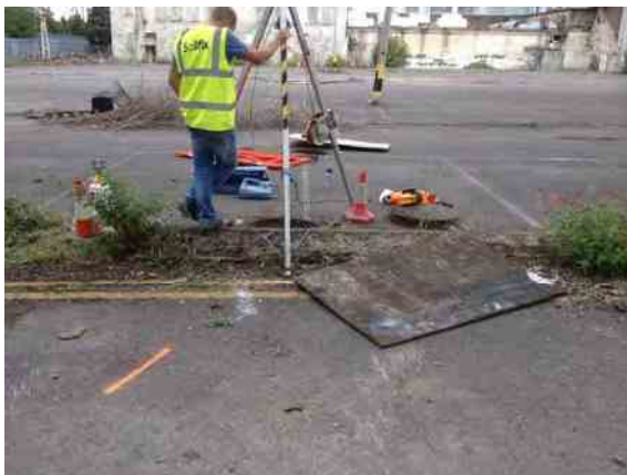
Topman during confined space entry
