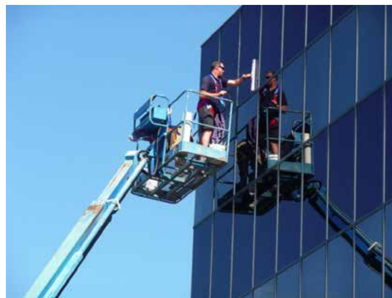
EXAMPLE OF CHERRY PICKER FACADE CLEANING
