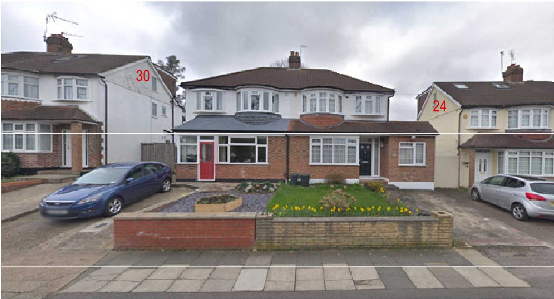
FRONT VIEW Showing gable end dormer extensions to number 24 Fore Street and 30 Fore Street
