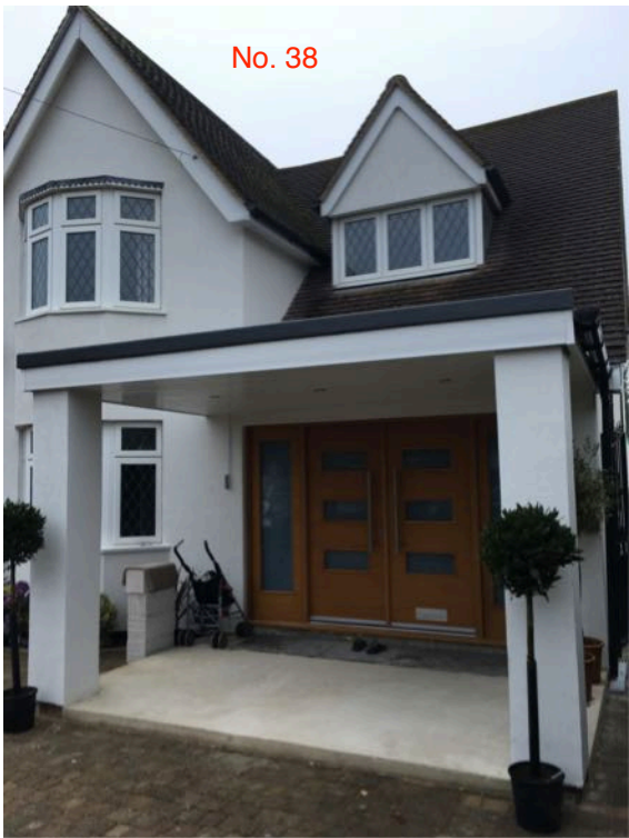
View from driveway of as built canopy
