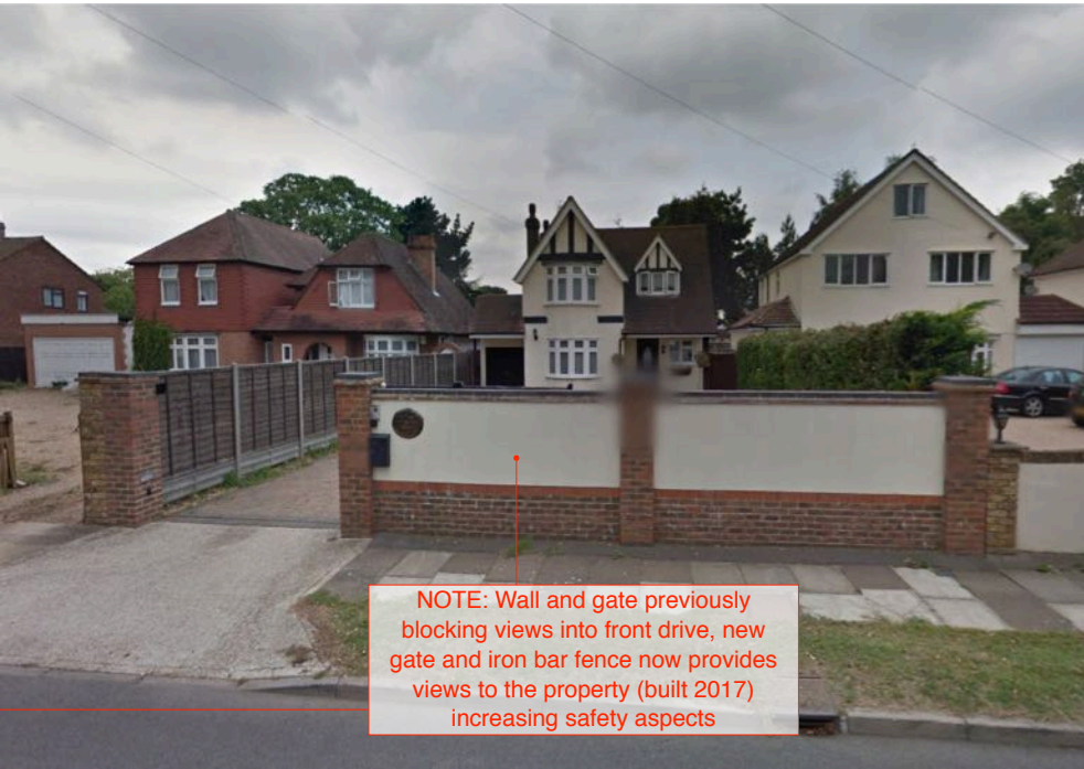
Historic view of the front elevation in 2014
