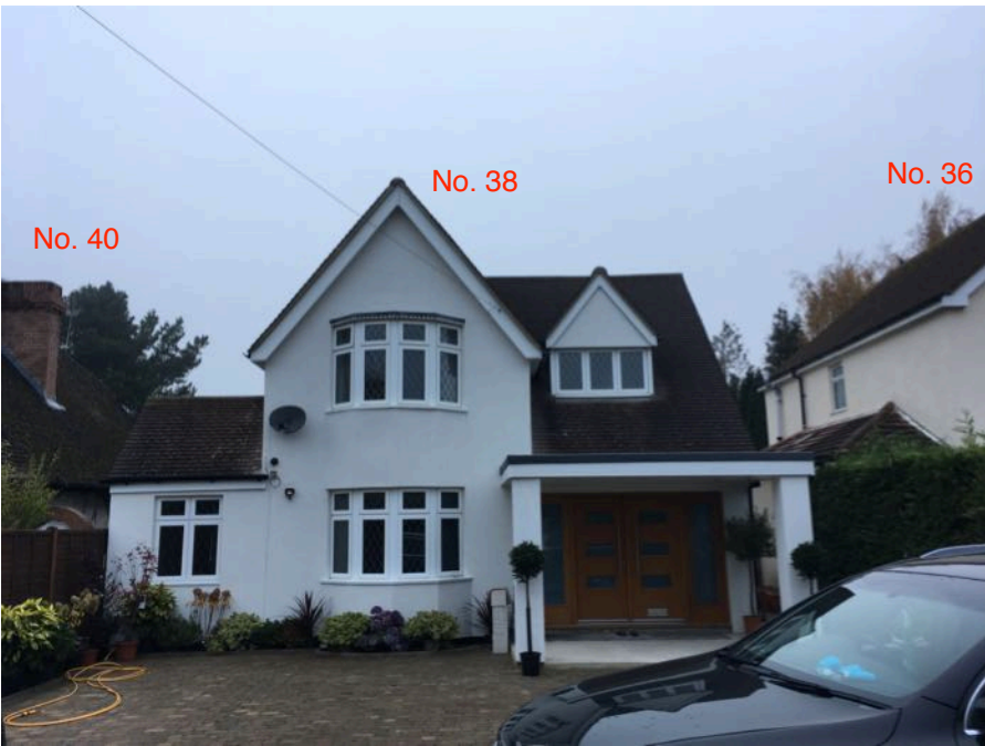
View from driveway of as built canopy
