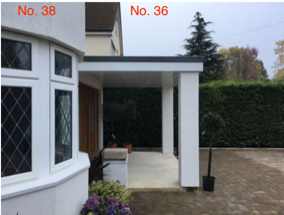
View of the as built canopy from the side
