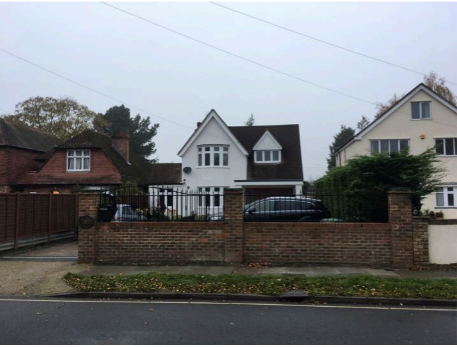
View of the front elevation in 2017 (Photo taken 15.11.17)
