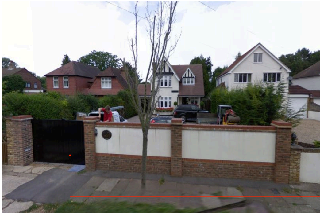
Historic view of the front elevation in 2008
