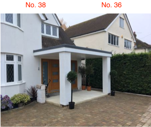
View of the as built canopy from the front
