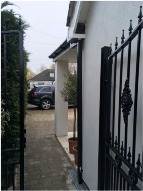
View from side alley of as built canopy
