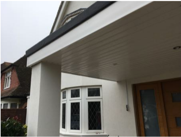
View of the underside of the as built canopy
