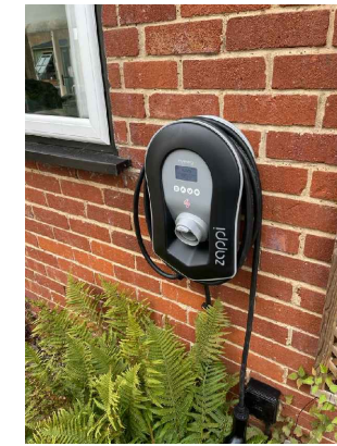
Zappi multiphase, car chargers With selectable power settings of 7kW and 22kW (6)
