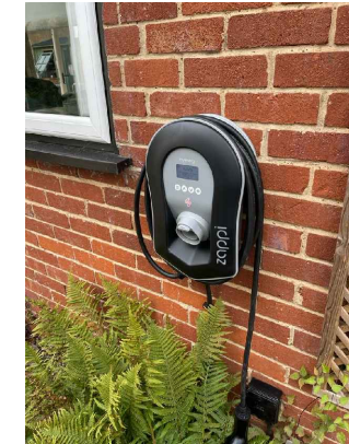
Zappi multiphase, car chargers With selectable power settings of 7kW and 22kW (6)
