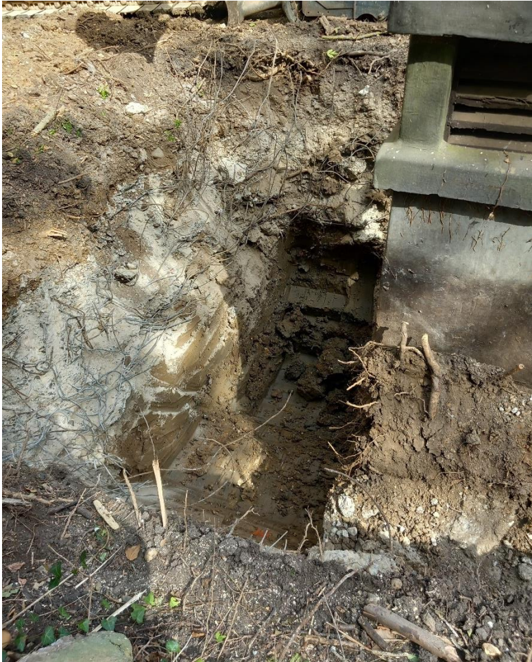
Image 2 mid-excavation section of Vent X2, showing upper concrete burster slab and clay layer below
