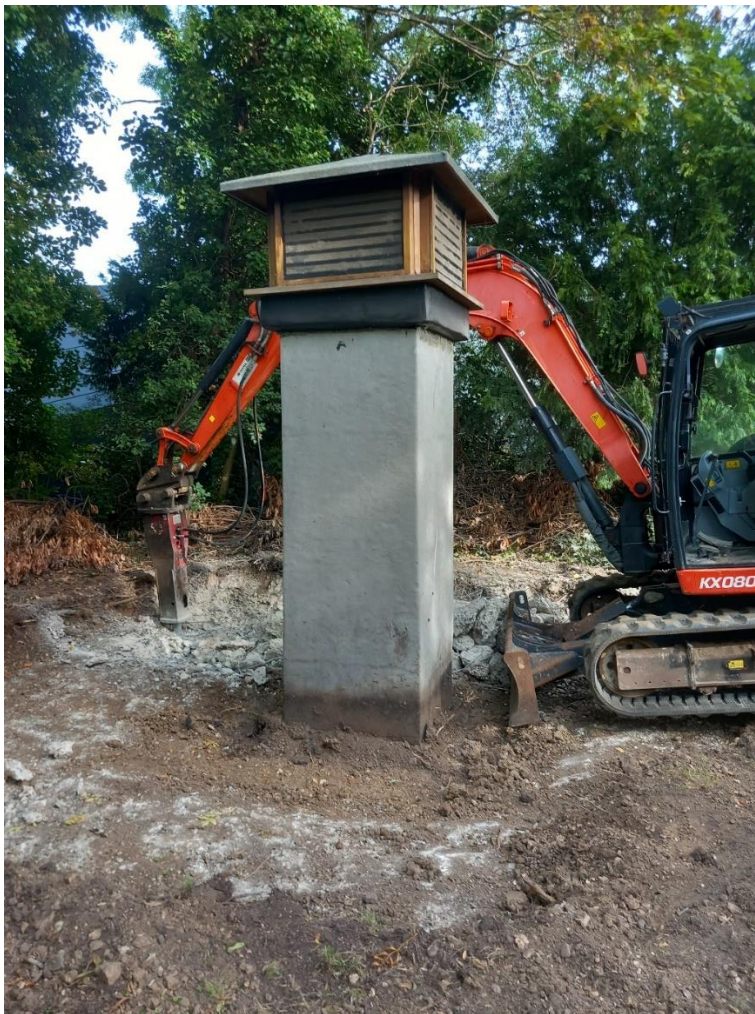
Image 1 the upper concrete burster slab being exposed near Vent X1 (looking NE)
