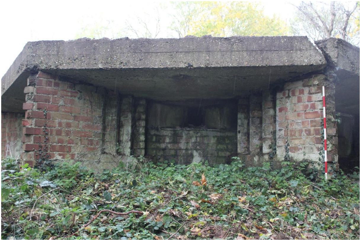
Image 5 the pillbox showing the brick 'spurs'(looking N)
