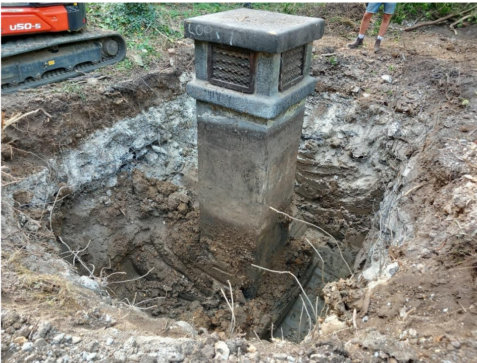
Image 3 mid-excavation view of Vent Y2, showing upper concrete burster slab and clay layer below
