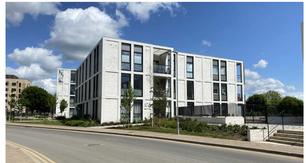
Photos of The Dice blocks on adjacent site where precast panel was changed to a metal panel due to technical and viability issues. A similar approach is proposed on this scheme with no compromise to design quality or built product.
