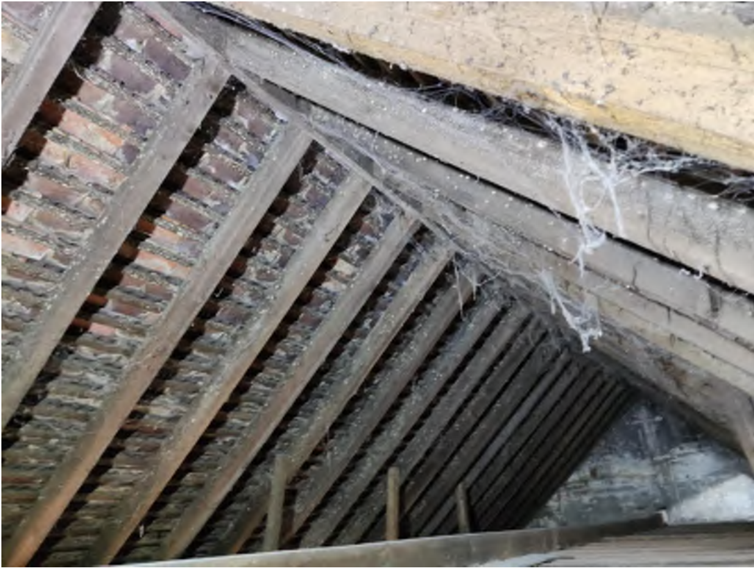
Photo 2: Roof Structure in good condition
