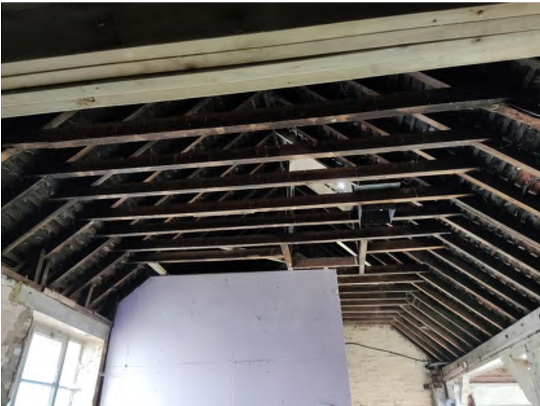
Photo 5: Roof Structure in good condition
