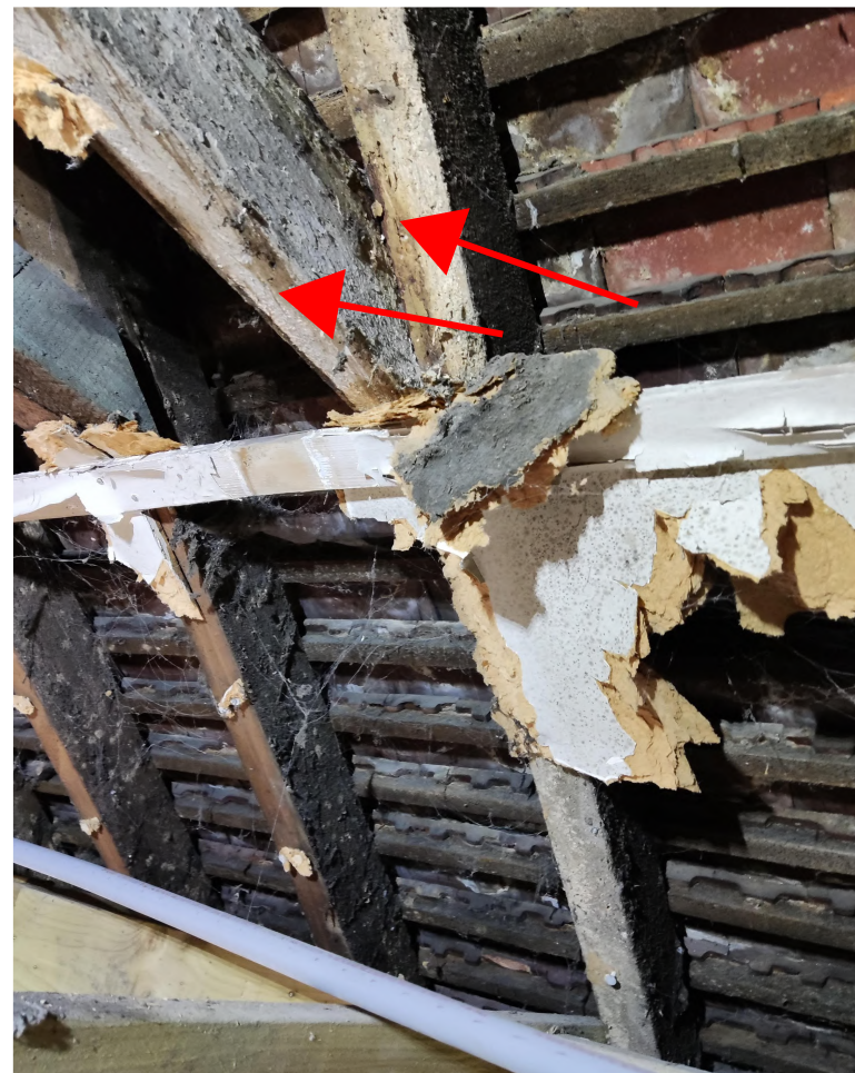
Roof Frame 29 decayed and should be fully replaced.
