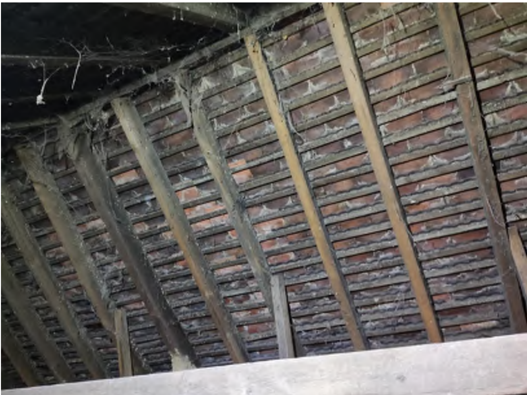
Photo 3: Roof Structure in good condition
