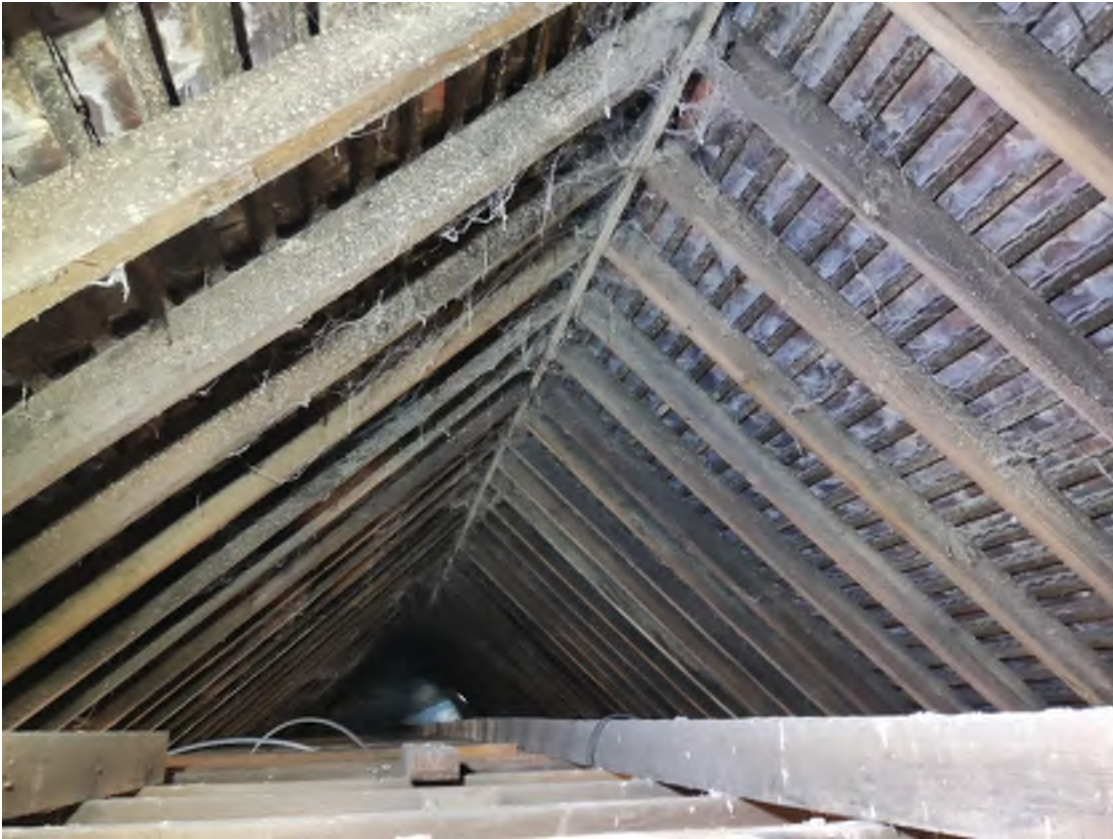
Photo 4: Roof Structure in good condition
