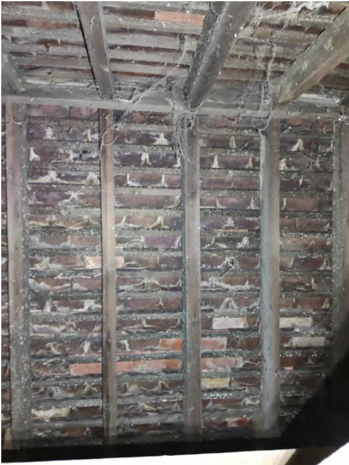
Photo 1: Roof Structure in good condition
