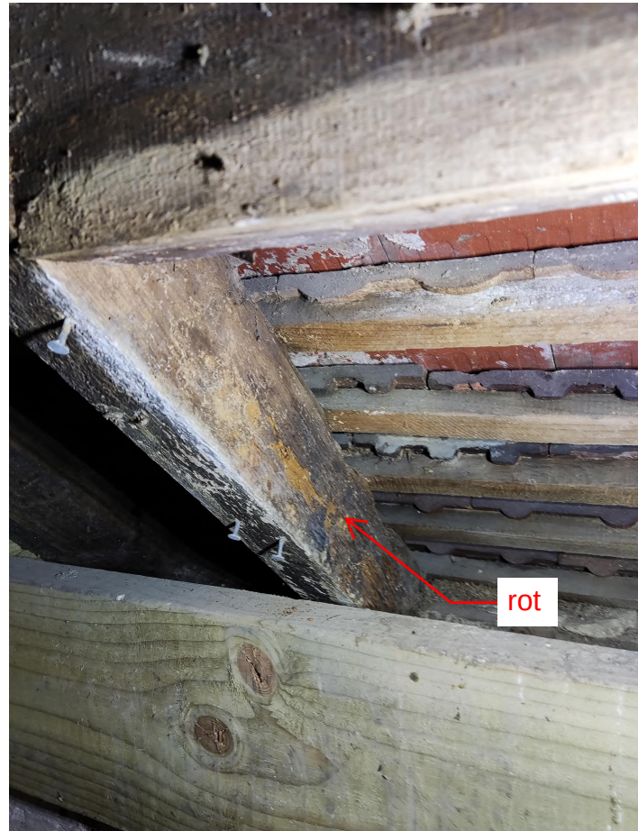
Roof Frame 40 decayed and should be replaced.
