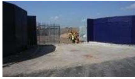
Typical St Modwen Homes site entrance gate
