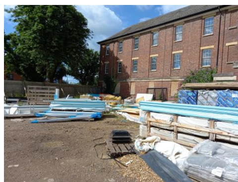
Rear of The Mons Building
