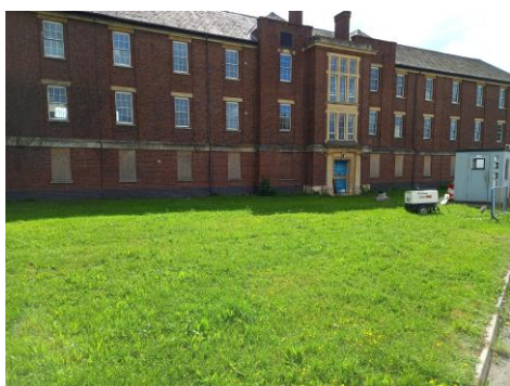
The Mons Building and surrounding lawns
