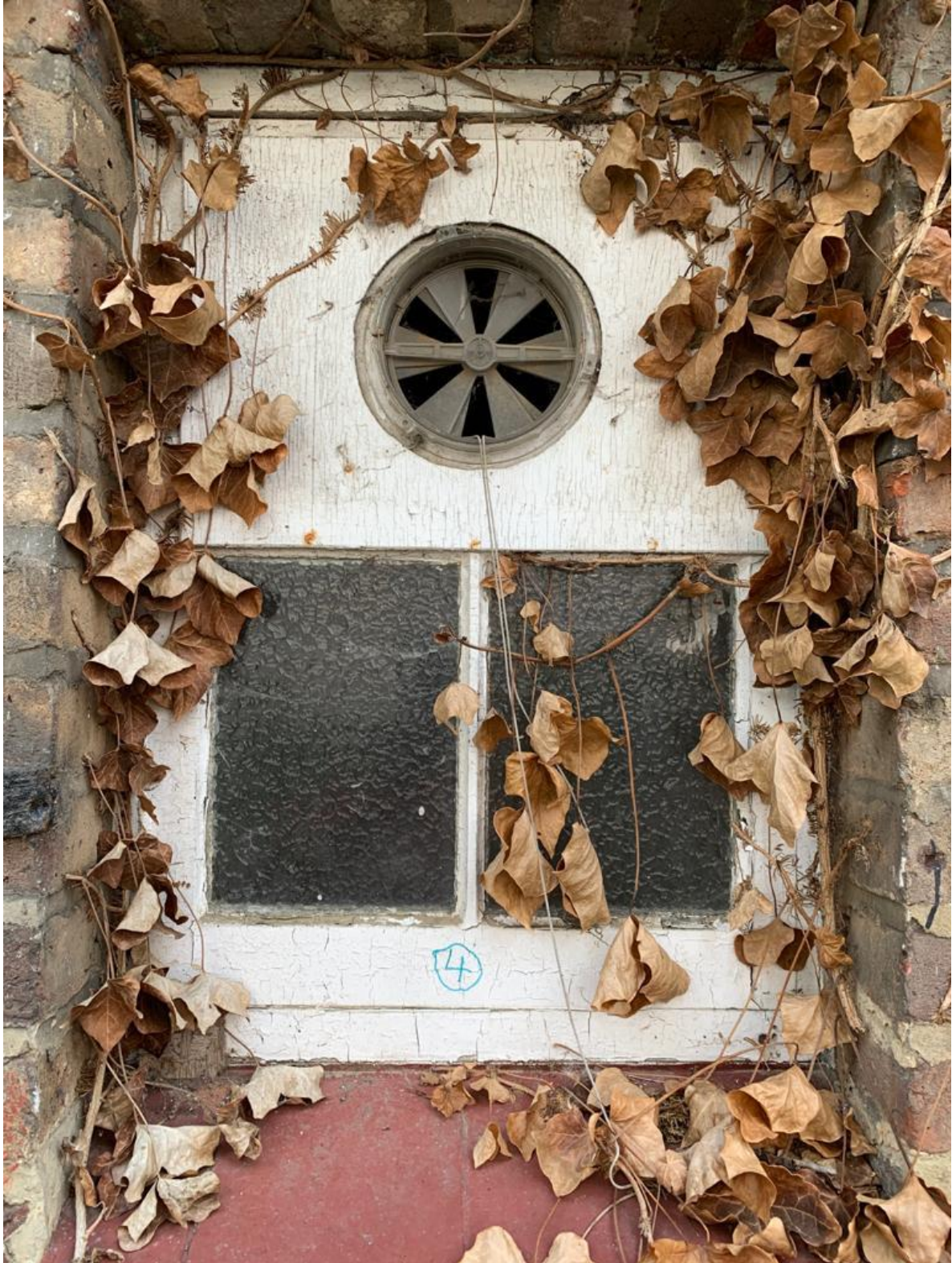
Window 4 (Timber) with vent
