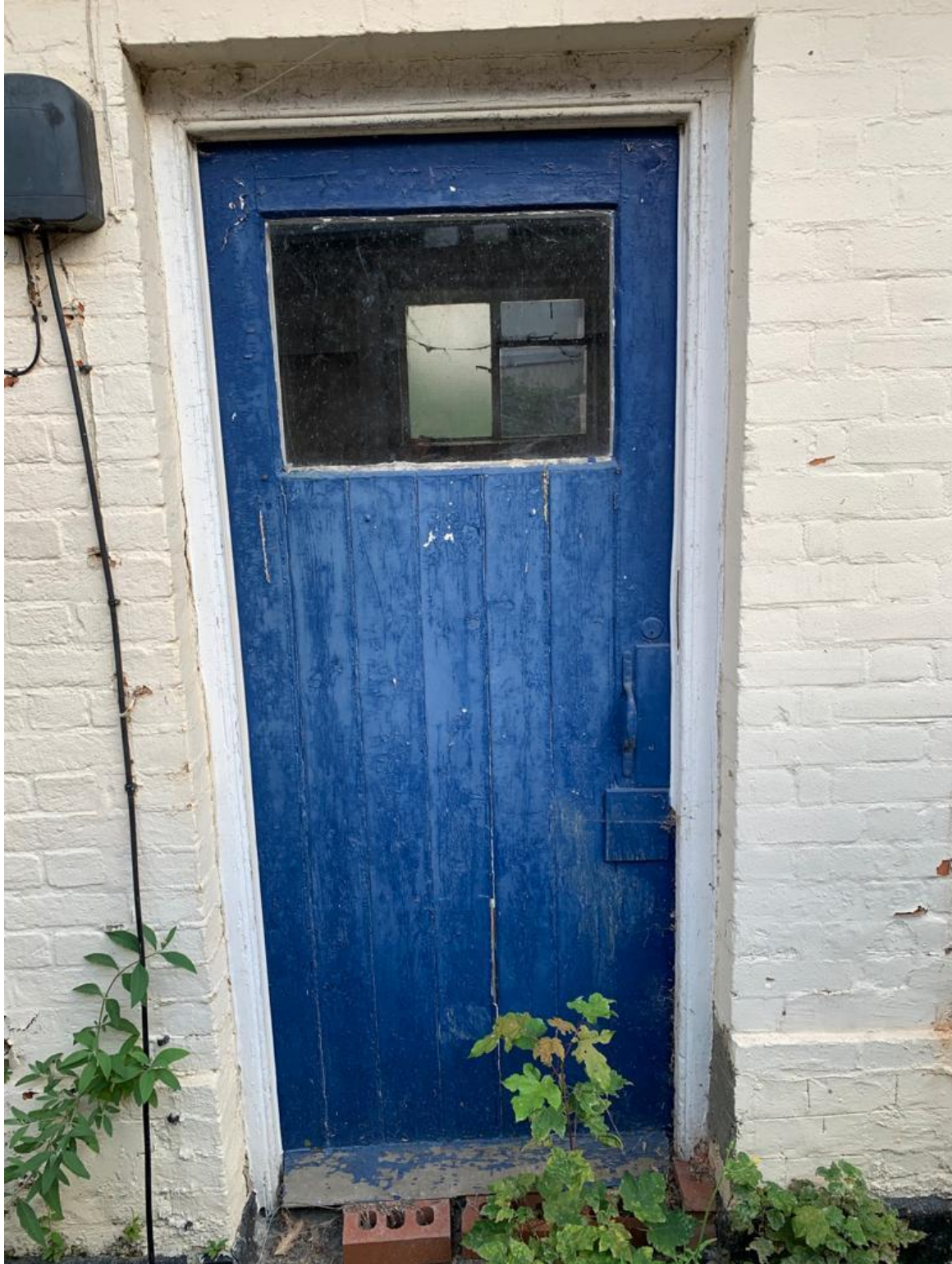
Timber Door to front / side
