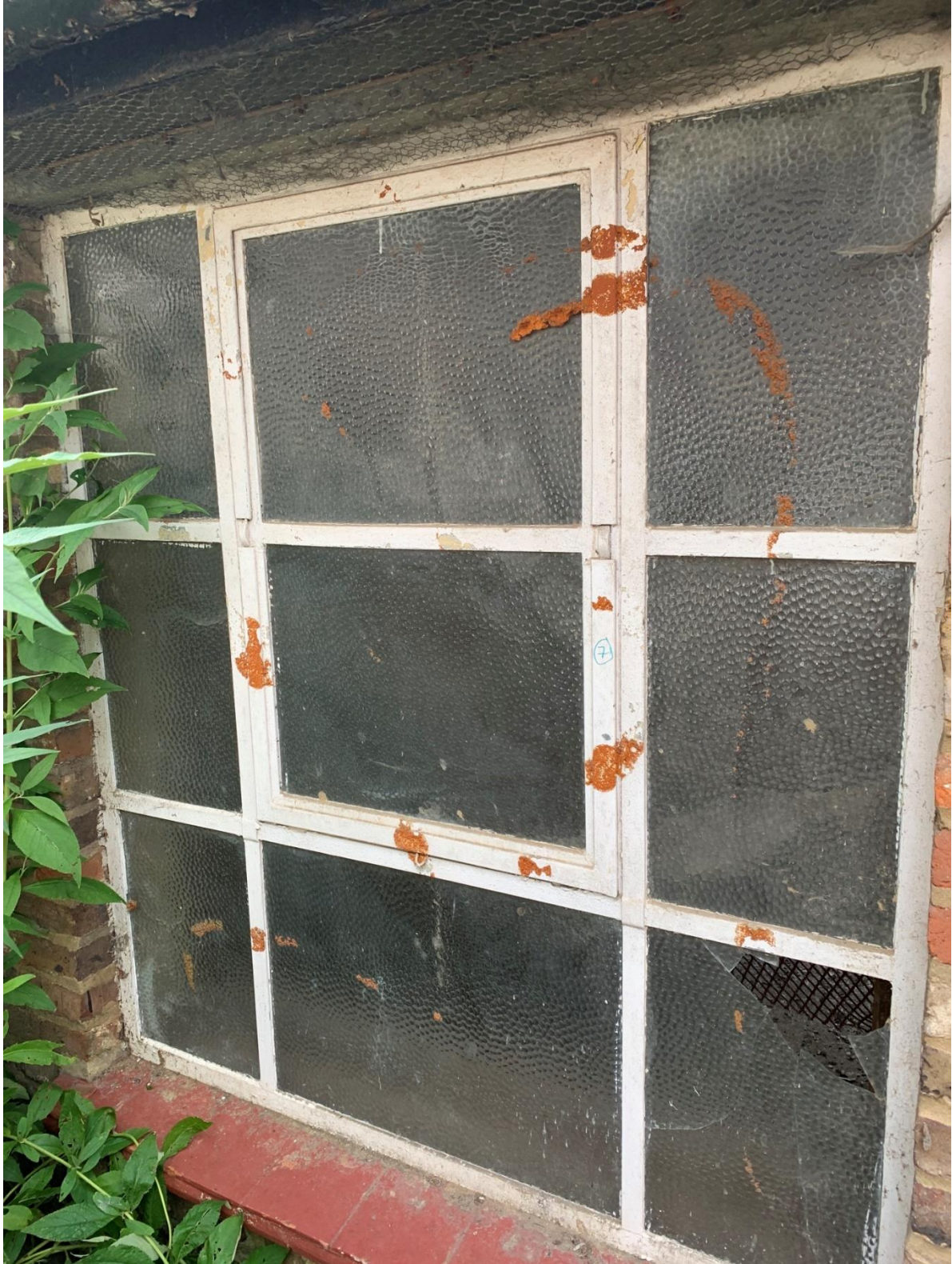
Window 7 (Crittall style / steel frame)
