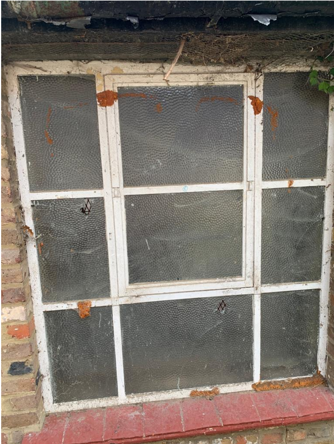
Window 8 (Crittall style / steel frame)
