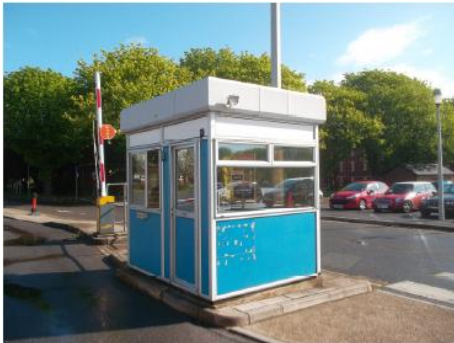
Security booth located off the site entrance
