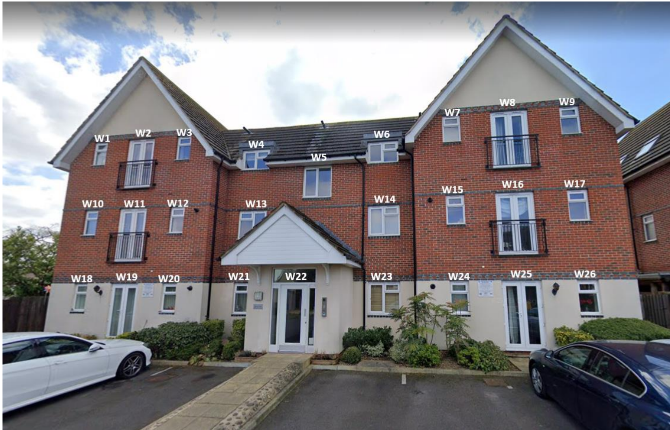
Figure 4.6: Assessed Windows at the Adjacent 555 and 557 Uxbridge Road
