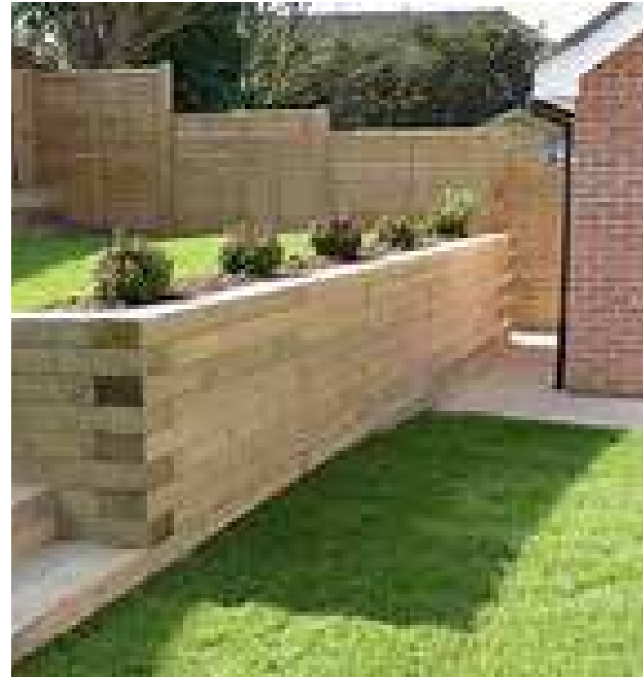
Timber Sleeper Retaining Wall
