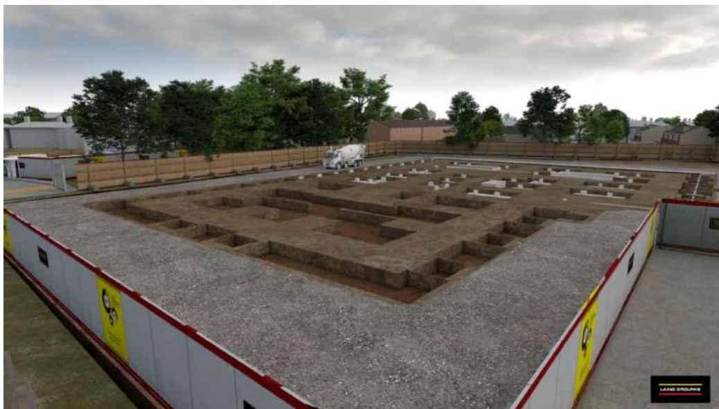
Figure 34 Foundations showing crane track around building footprint
