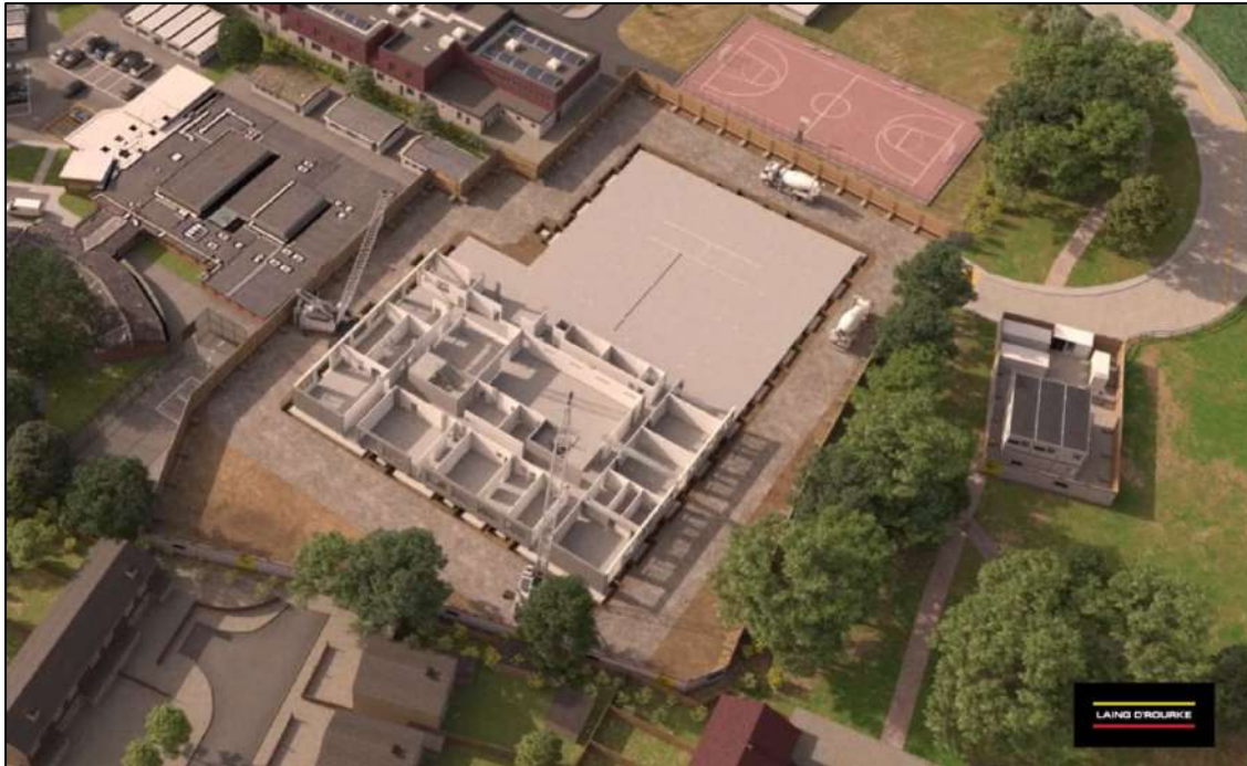
Figure 35 Crawler cranes constructing frame and internal walls (Smart wall)
