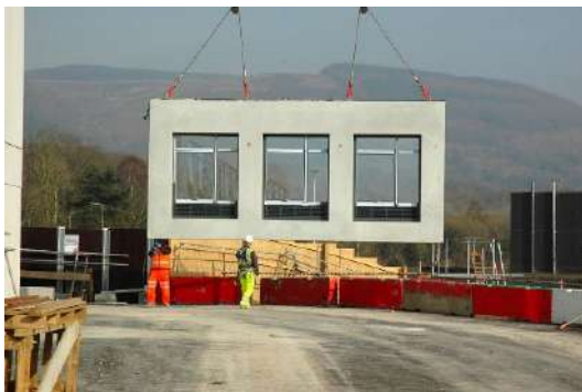
Figure 27 Cladding panels installed
