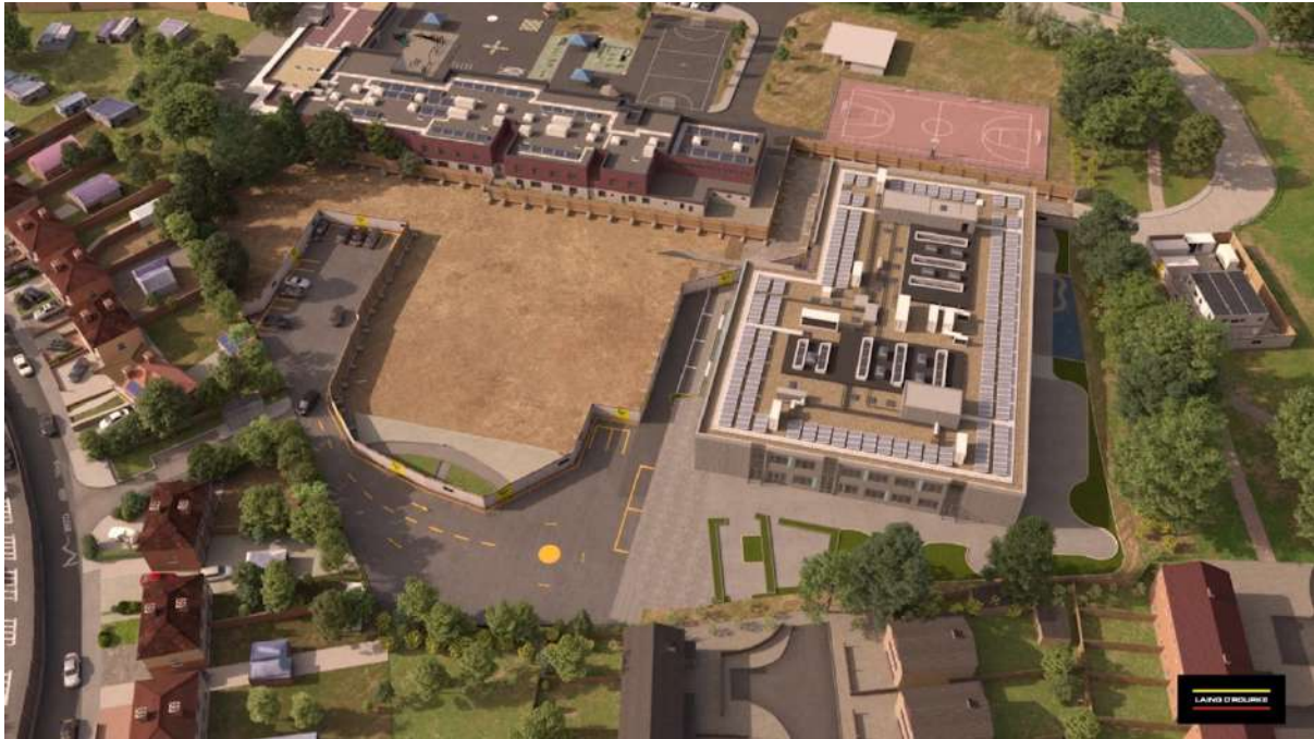
Figure 30 New school operational & start of demolition/landscaping
