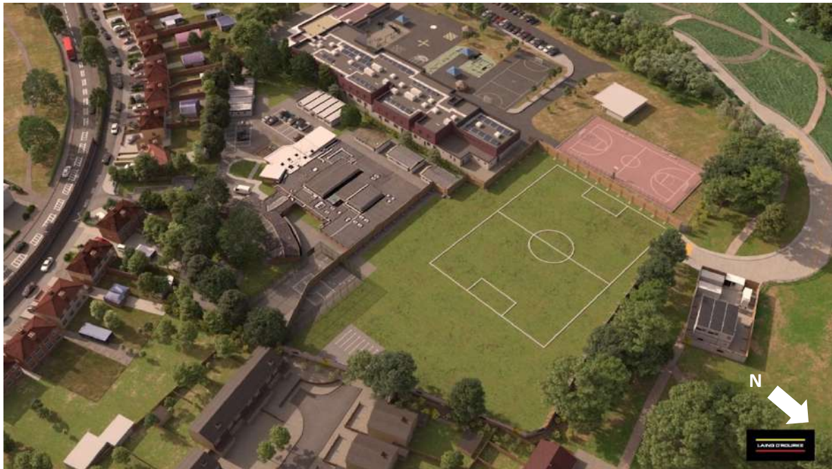
Figure 24 Weeks 1-5 Enabling Works
