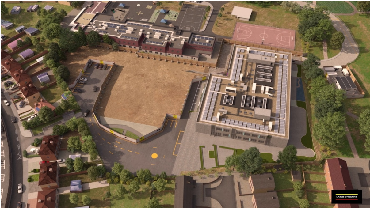
Figure 31 New school operational & start of demolition/landscaping
