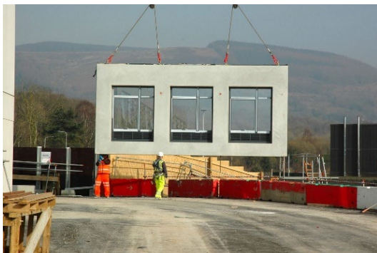
Figure 28 Cladding panels installed
