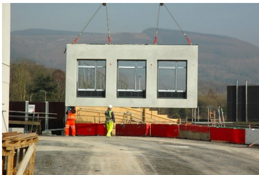
Figure 27 Cladding panels installed
