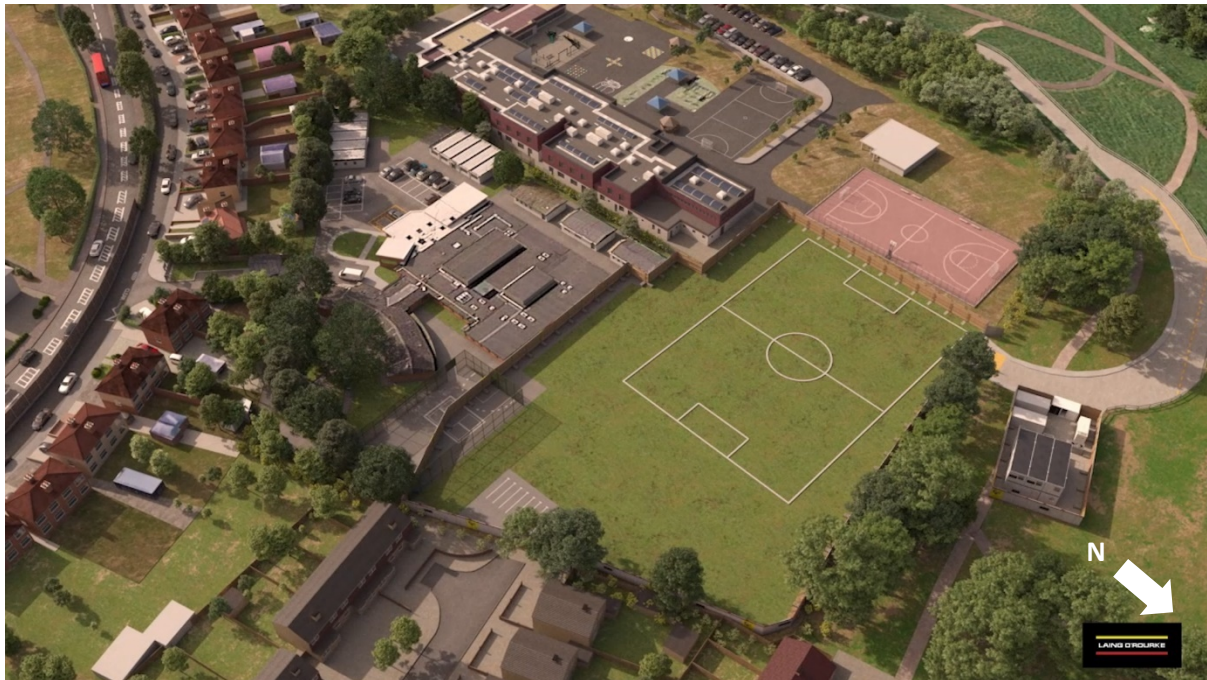
Figure 24 Weeks 1-5 Enabling Works
