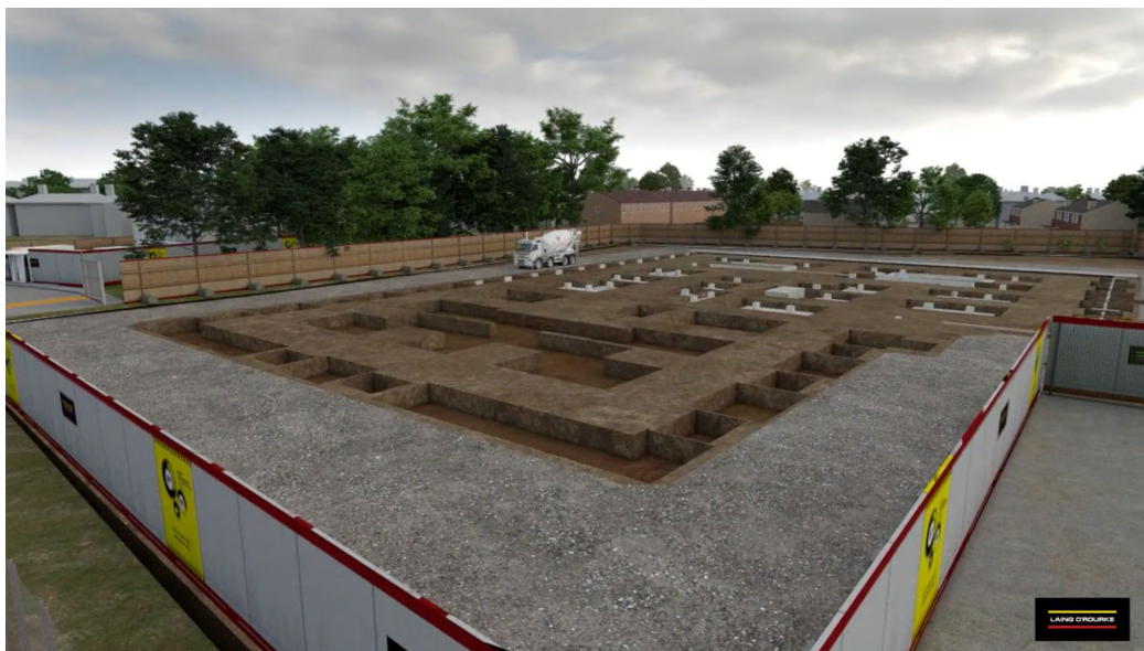
Figure 34 Foundations showing crane track around building footprint
