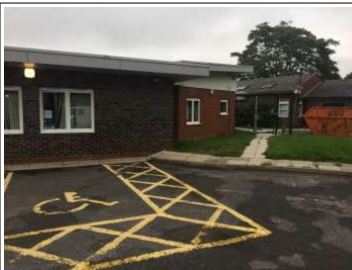
Main school building
