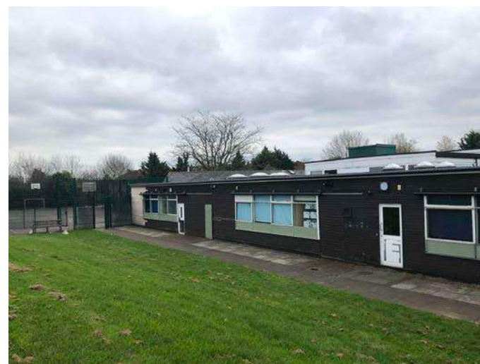
10. Existing school building.
