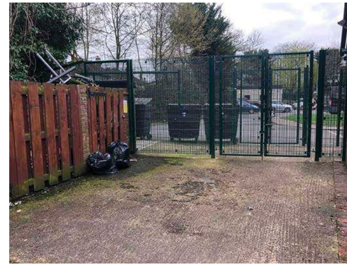
12. Existing refuse area towards main vehicular route.
