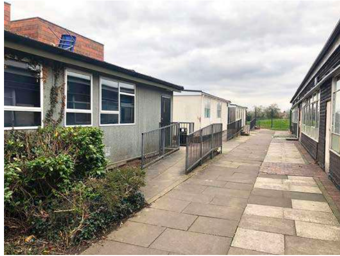
7. Existing school building and external pre-fab classroom.
