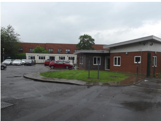
5 Range of recent, single storey and temporary school buildings located towards the central western section of the site, view west
