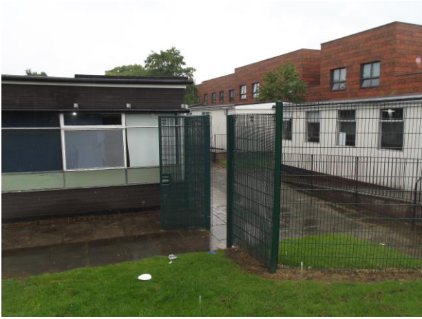
7 Range of recent, single storey and temporary school buildings located towards the central western section of the site, view south
