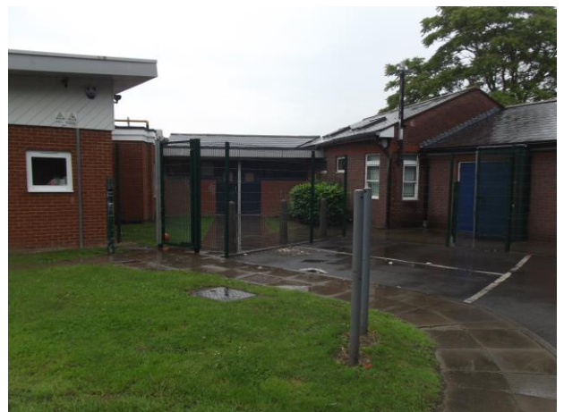
6 Recent school building located towards the central western section of the site, and which comprises a modern, single storey structure, view north-east
