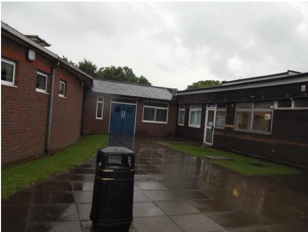
3 Main school building located towards the centre of the site, and which comprises a modern, single storey structure, view north
