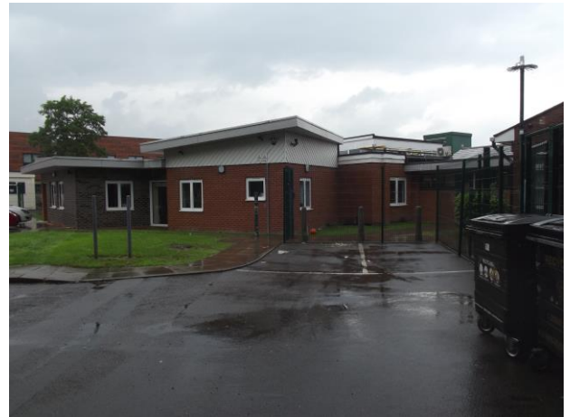
4 Recent school building located towards the central western section of the site, and which comprises a modern, single storey structure, view north-west
