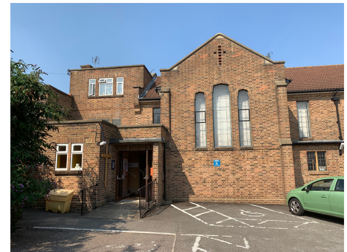
view of the South transept window and existing side entrance
