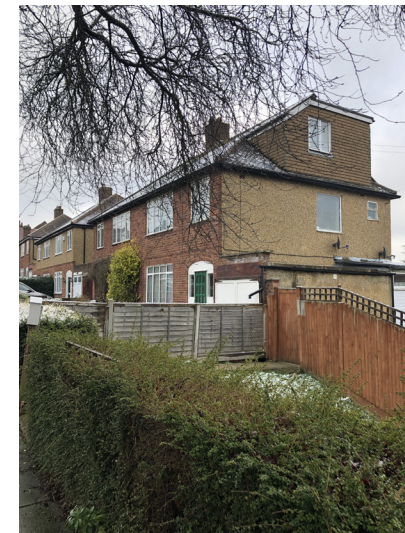
view of neighbouring house on North side
