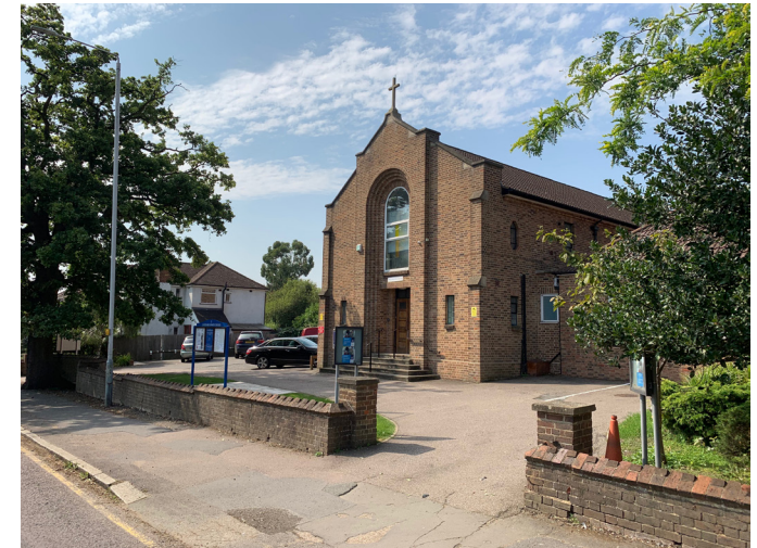
existing view of church from the North on Joel Street
