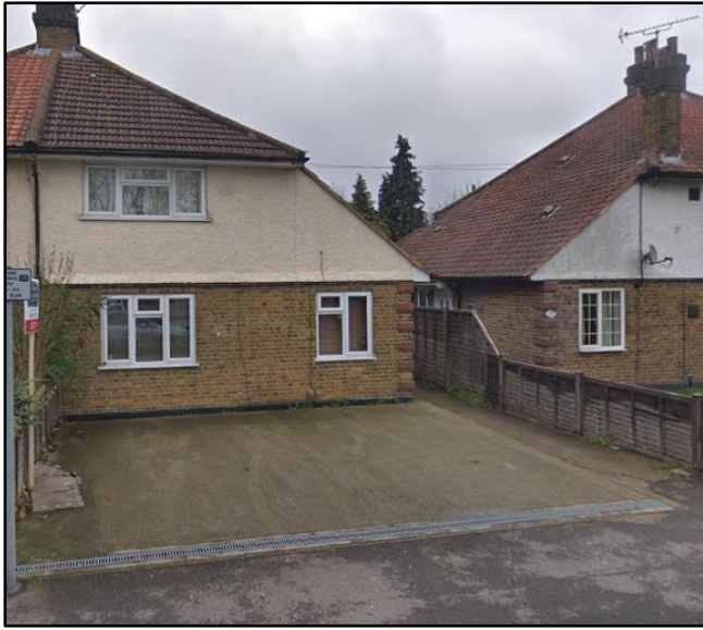
Figure 4 – Hard surfaced front curtilage at No. 101 The Greenway.
