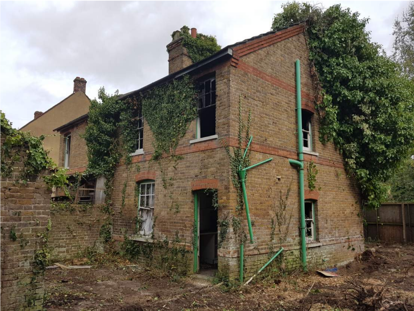
General view, showing existing building, looking East
