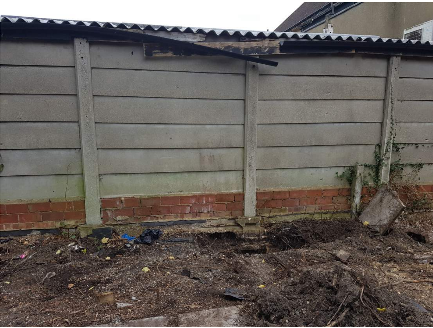
TRIAL PIT 7 - Showing Boundary with No 19/21
