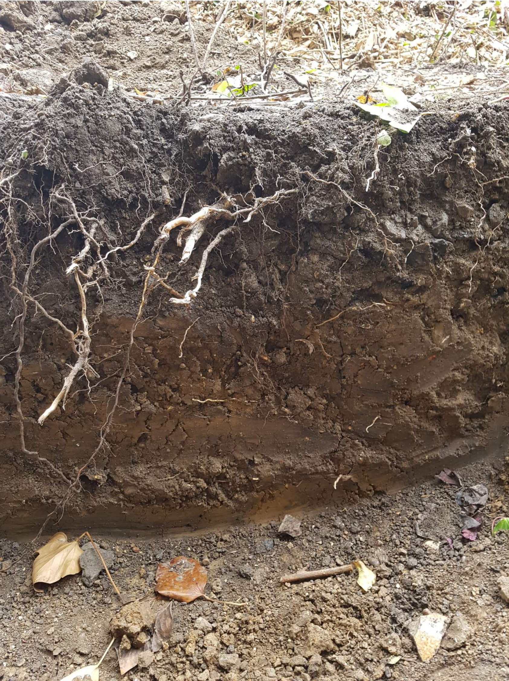
TRIAL PIT 1 - Showing made ground over clay
