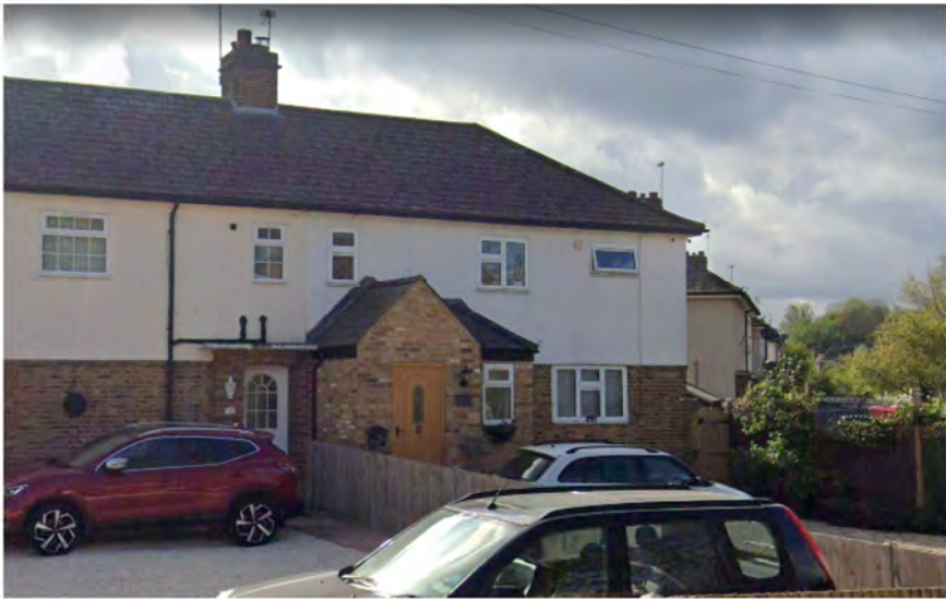
No.16 Priory Avenue, Porch
