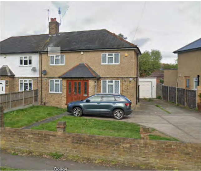
No.9 Priory Avenue, Porch
