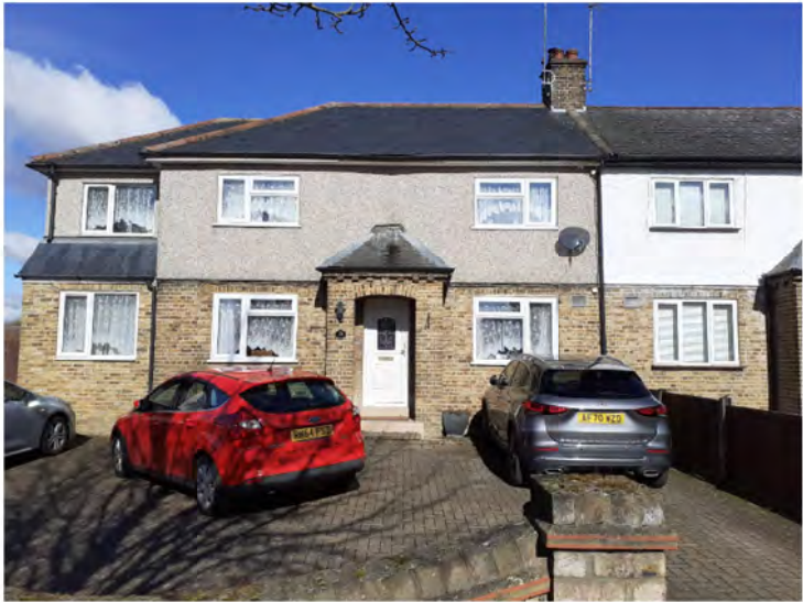
No.23 Priory Avenue, Existing Front Porch / Driveway
