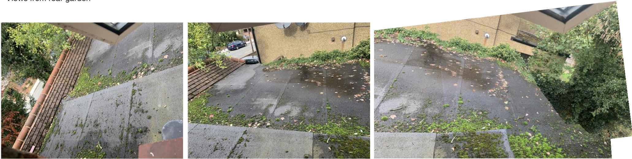
Views from first floor window looking towards the garage close to neighbour's property
