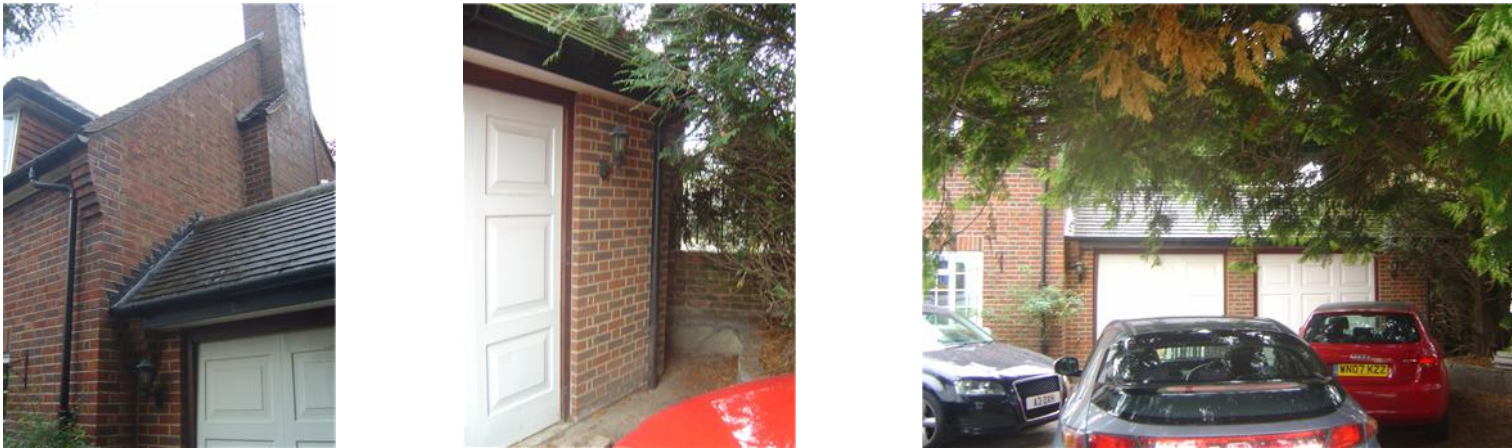
Views from front drive looking towards the garage
