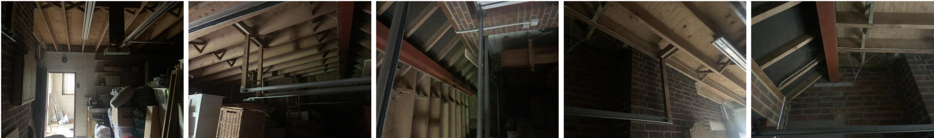
Views from the garage
