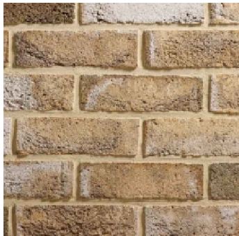
DETAIL OF BRICK WALLS OF CYCLE STORAGE AND REFUSE STORAGE
