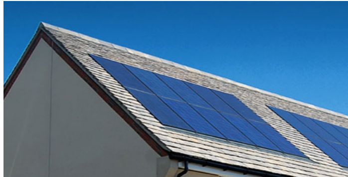
Figure 9: Typical PV installation to pitched roof
