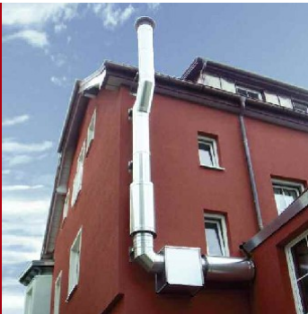
Outdoor installation with wall bracket (accessories).
