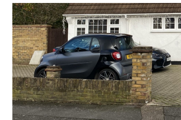
Low level boundary wall at No.14
