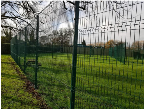
New fence TYPE A 3m green wire
