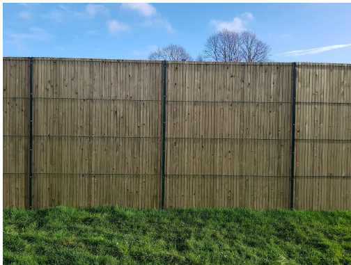
New fence TYPE B 3m green wire with timber slat inserts
