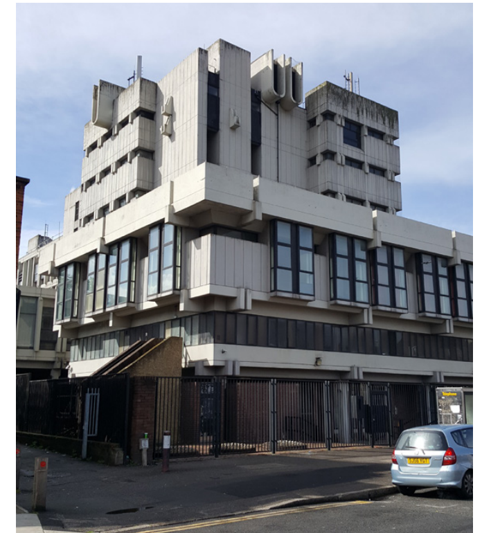
6. View of British Telecom building opposite site on East Avenue.
