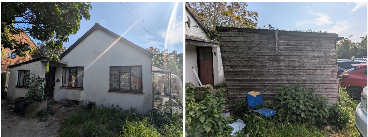
Figure 4. View of the bungalow and shed within the residential curtilage
