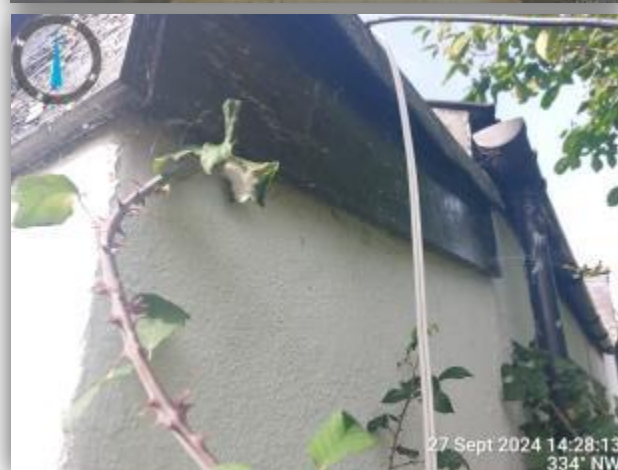
Gap under fascia board on east elevation.
