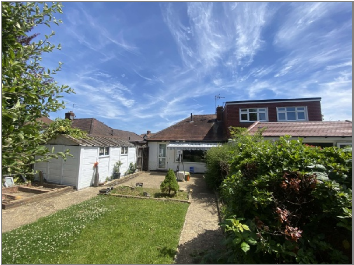
view - rear neighbouring elevation
