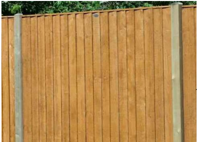
Proposed 6ftx6ft closeboard timber fence panels with concrete post and gravel board timber fence with 2m height for boundary treatment between Flat A&B gardens.
