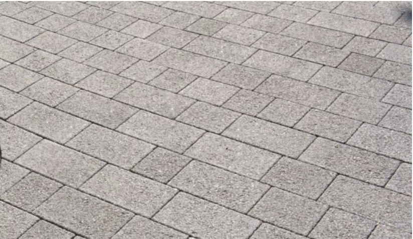
Example of permeable driveway - car parking spaces
